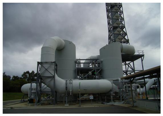
The majority of the gas extraction comes from the Bioreactor and Membrane Tanks in Stage 1 and in the Ultimate development. Many odour control facilities do not extract "odour" from the aerated sections of the tankage but the close location of the WRP to housing (as close as 100 m from the drawing below) makes this understandable.
