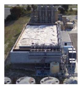
Often the submerged membranes are included at the end of the tank (as shown above and below), rather than a separate membrane tank, which lowers both capital and operating costs (no extra pumps). In other cases pressure membranes are external to the bioreactor.
