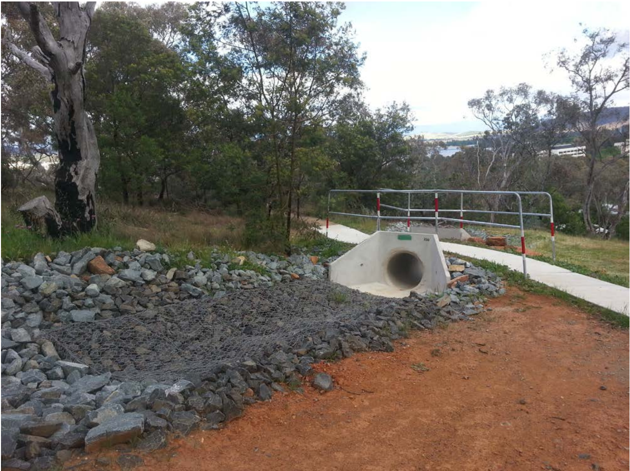
Figure 2 Discharge dissipater example
