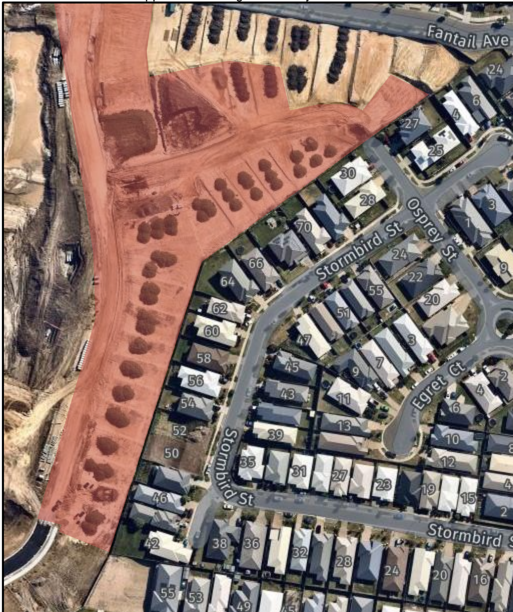
Picture 1: Aerial View of the Site (Image Source: Nearmap.com 25 th April 2021) Approximate Stage Boundary shaded red
