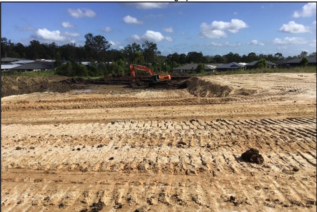
Picture 5: View of Filling Operations
