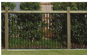
Timber & infill 'pool fencing'
