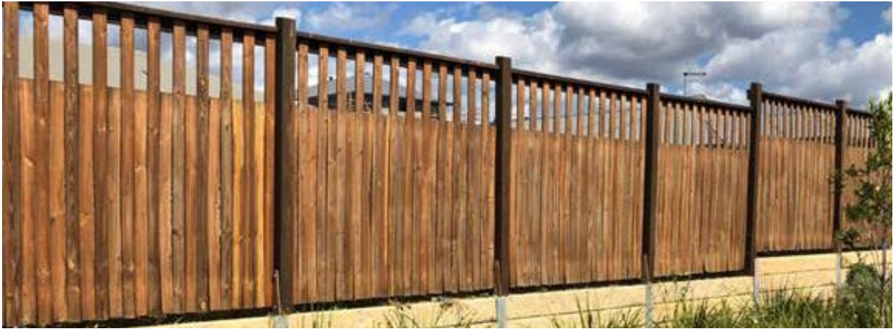
Figure 4: Typical Flagstone fencing type
