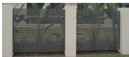
Street frontage / secondary street frontage masonry fence
