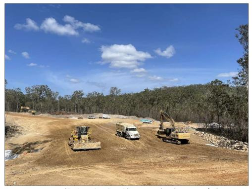
Figure 4 – Compactor working in conjunction with water truck and excavator. (Taken 19.11.2020)
