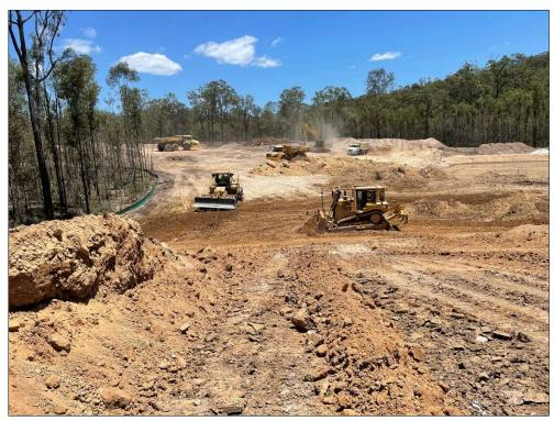
Figure 1 – Heavy machinery placing and spreading out fill. (Taken 05.11.2020)
