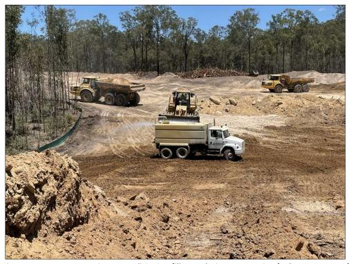
Figure 2 – Water cart moisture conditioning fill area during compaction (Taken 05.11.2020)
