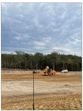
Figure 6 – Pad foot roller and water truck working fill pad. (Taken 13.11.2020)
