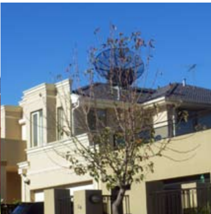
EXPOSED AND OVERSIZED SERVICES ON ROOF
