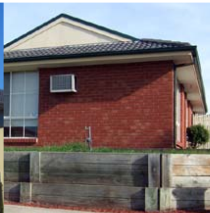
VISIBLE CONDENSER UNITS TO THE STREET FRONT
