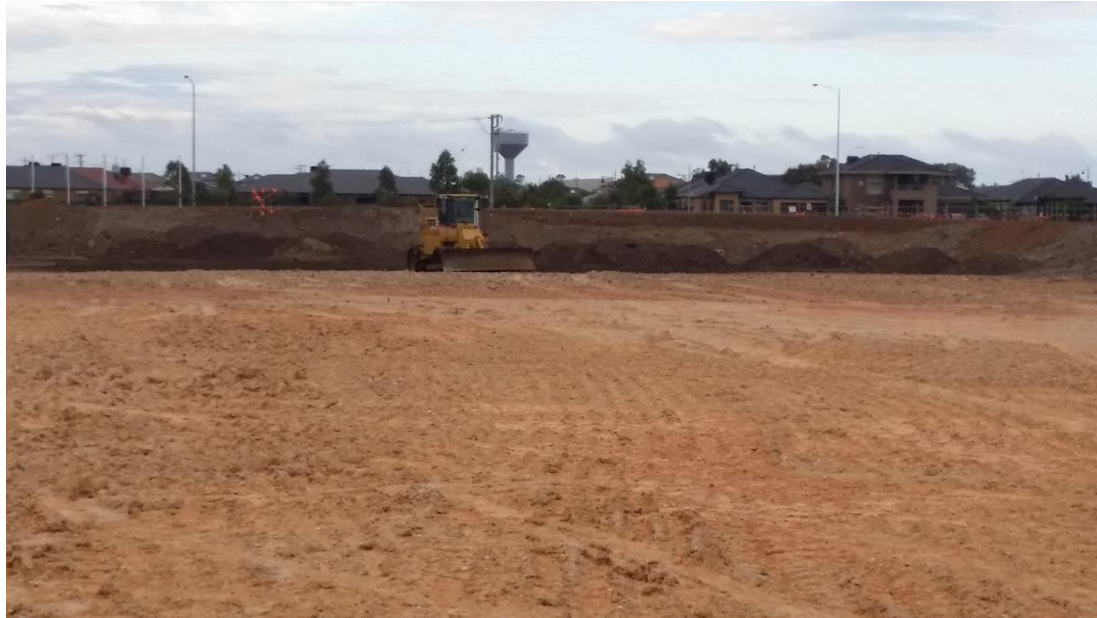
Stage 4: Placing of layer 1 material in grid N2 (E) and O2
