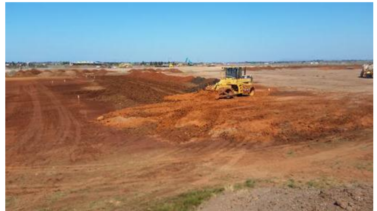
Compactor placing layer 1 - column D (east-south-east) and E (west-north-west).
