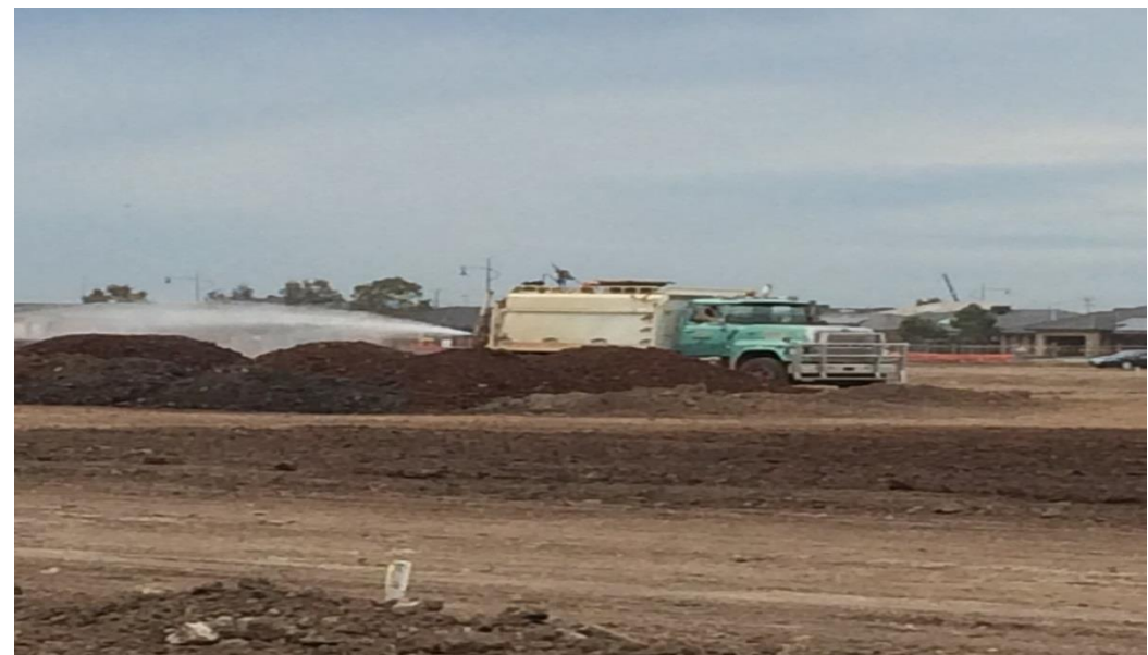
Water cart moisture conditioning the stockpile
