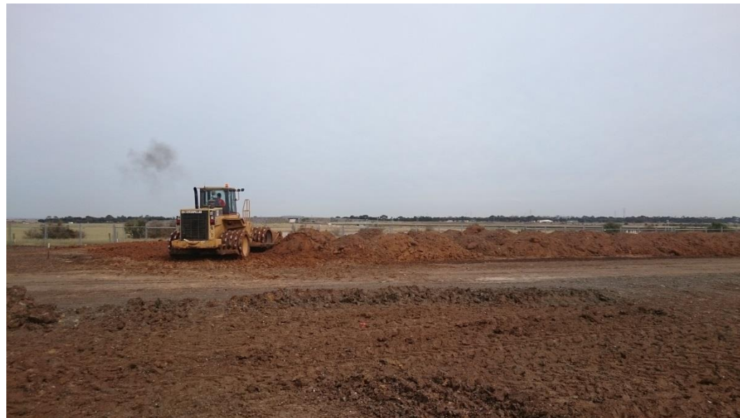
Compactor on layer 3 in grid A5 and A6
