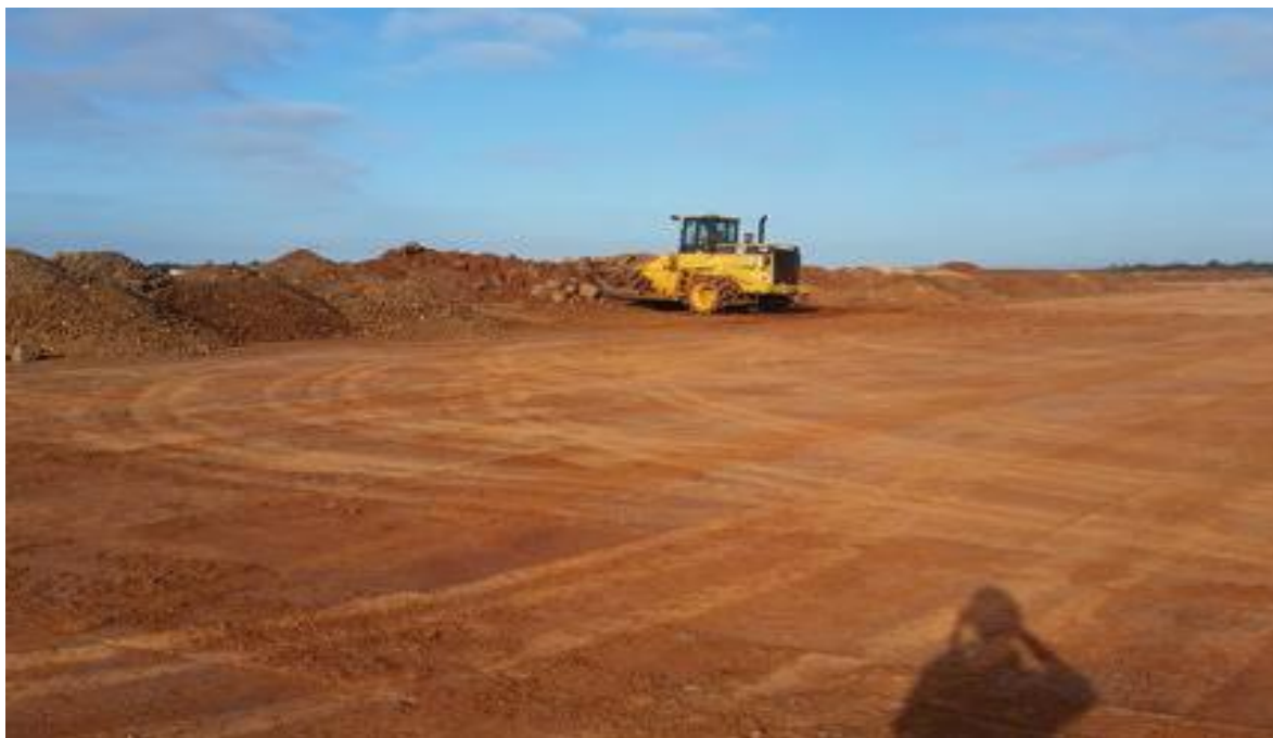
Compactor pushing-out boulders - F4 (south-south-west).
