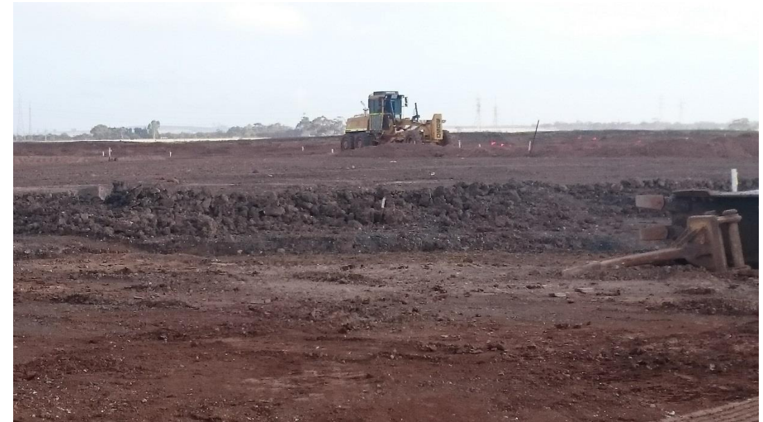
Stage 1: grader being used in grid N1, N2, O1 and O2
