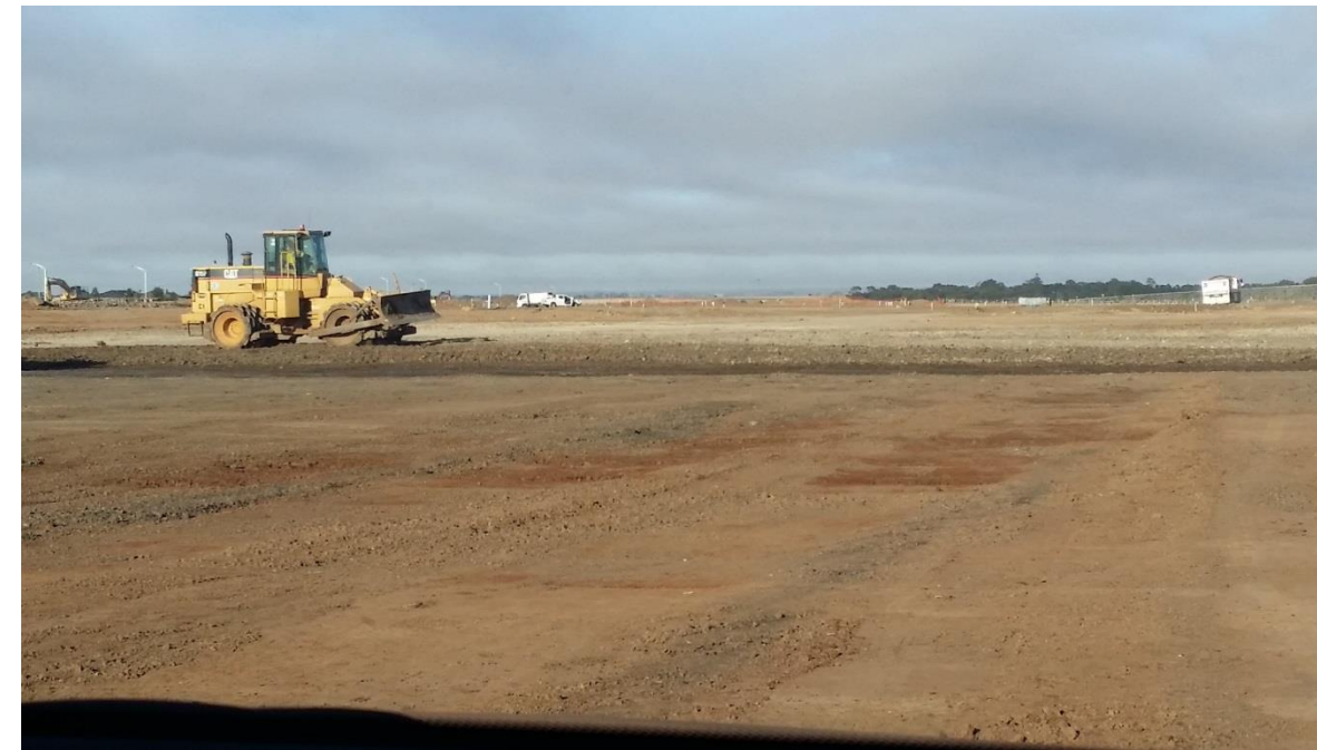
Stage 4: Compaction of layer 1 material placed in grid N4 and N5
