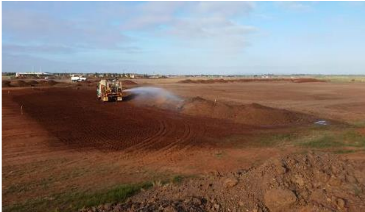
Water Cart moisture conditioning - column D (east-south-east) and E (west-north-west).
