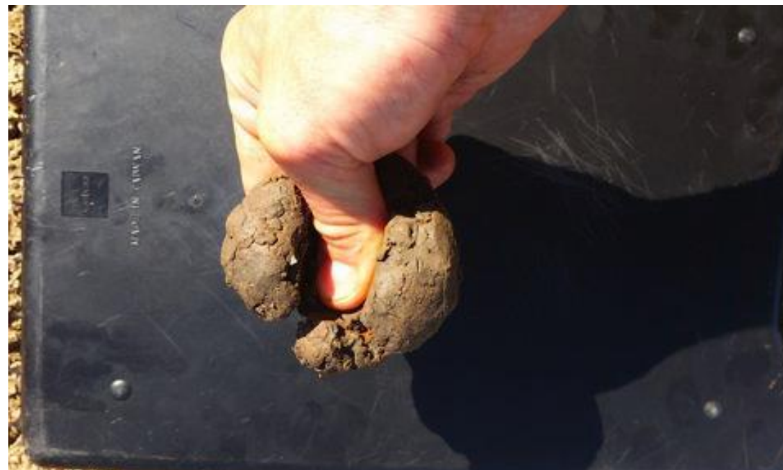
Layer 1 moisture condition assessed - E4 (north-north-east), F4 (north-north-east), and G4 (west-north-west)
