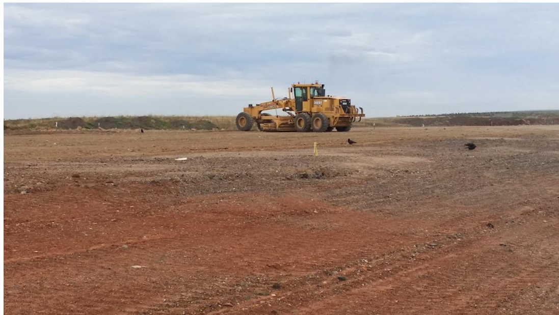
Stage 3: Grading to RL's in grid C5 (N), C6 (S), D5 (N), D6 (S), E5 (NW) and E6 (SW)
