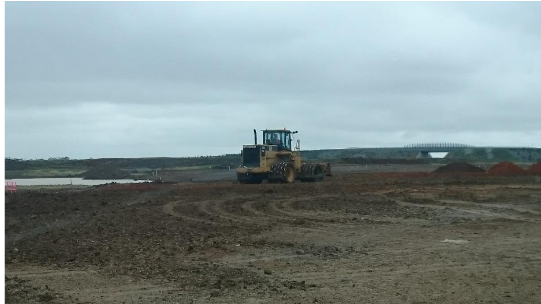
Stage 3: Compactor placing material as part of layer 3 and layer 4 (refer to Stage 3 site plan above)
