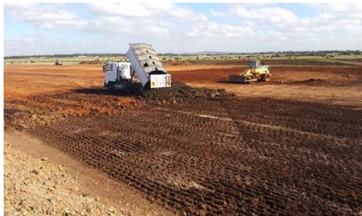
Dump Truck (tandem) unloading St Albans fill- G4 (north-west).
