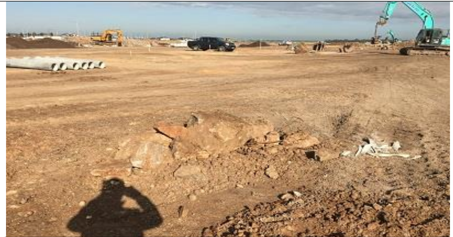
Photo 2 – Looking West From G6: Oversize which was removed from grid sections G6
