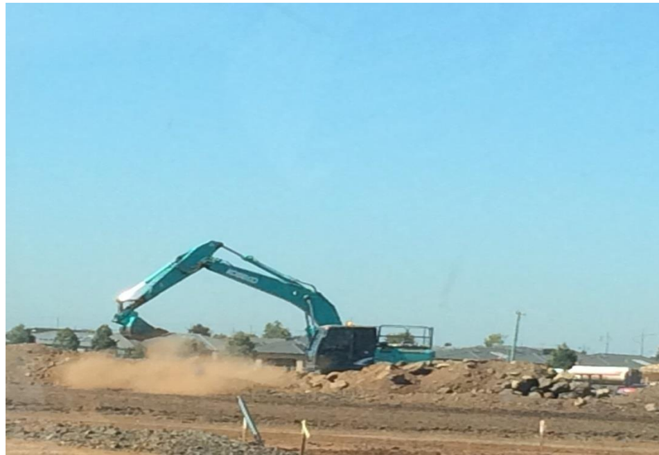
Excavator sieving boulders
