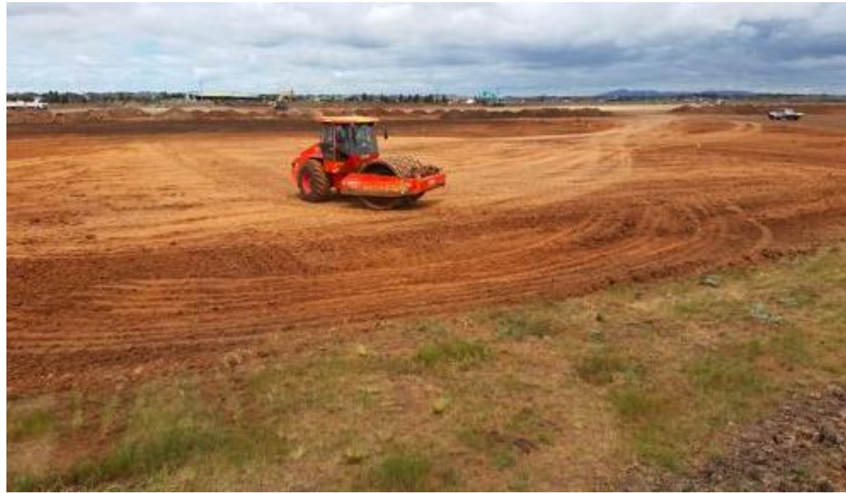
Padfoot Roller compacting layer 1 – E5 (east)/E6 (south-south-east)/F5 (west-north-west)/F6(west-south-west).
