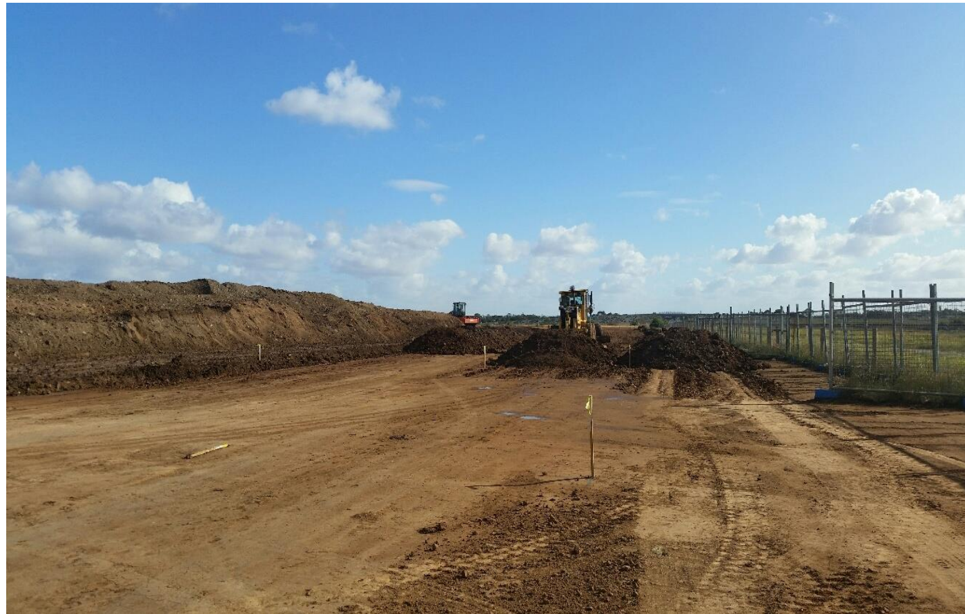
3. Material placement on grid D6
