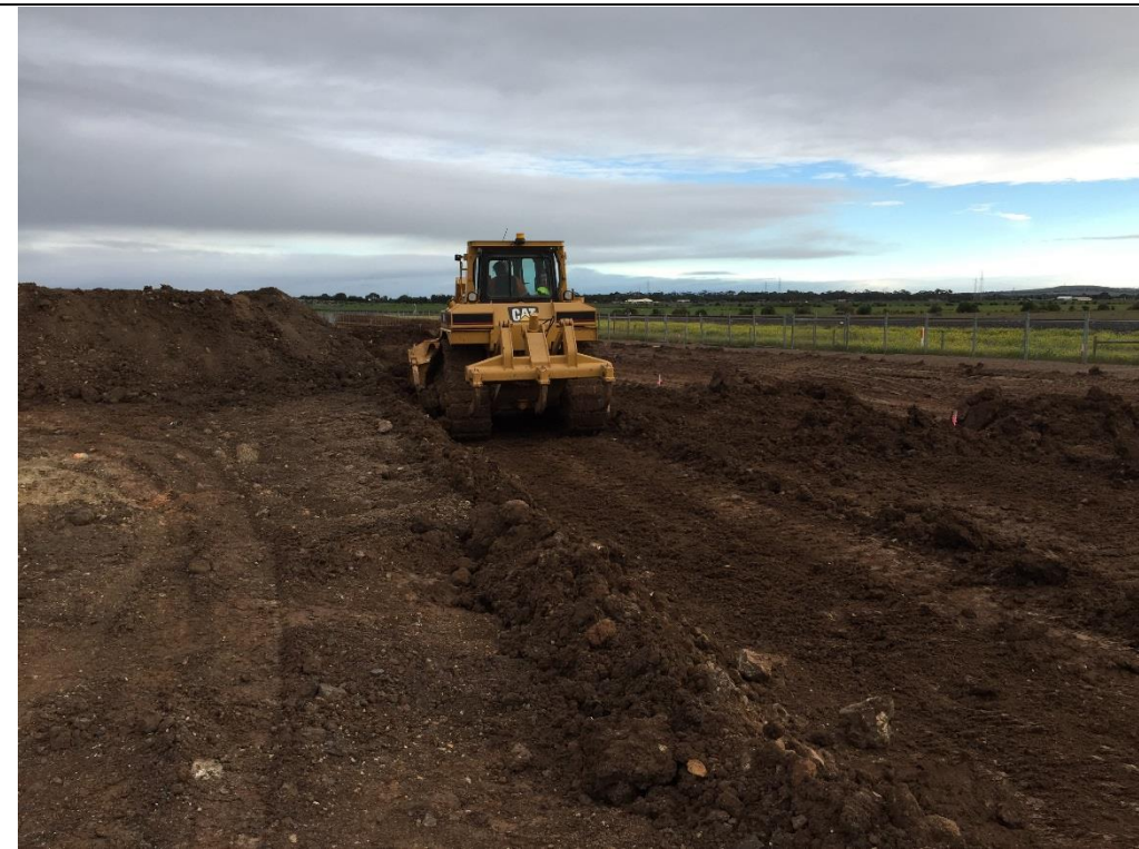
Stage 3: Dozers placing Layer 1 in grid B6, C6, D6
