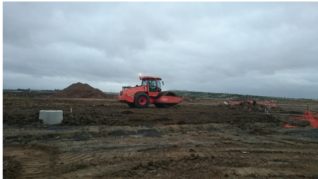
Stage 3: Compactor placing material as part of layer 3 and layer 4 (refer to Stage 3 site plan above)
