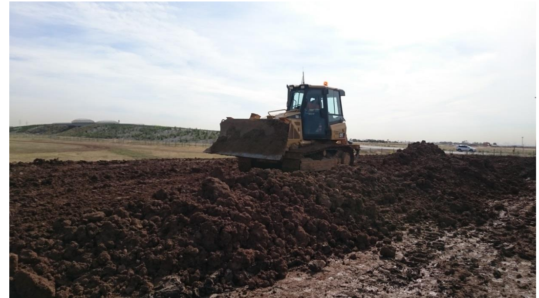
Stage 1: pad foot roller used on layer 8 in grid O2
