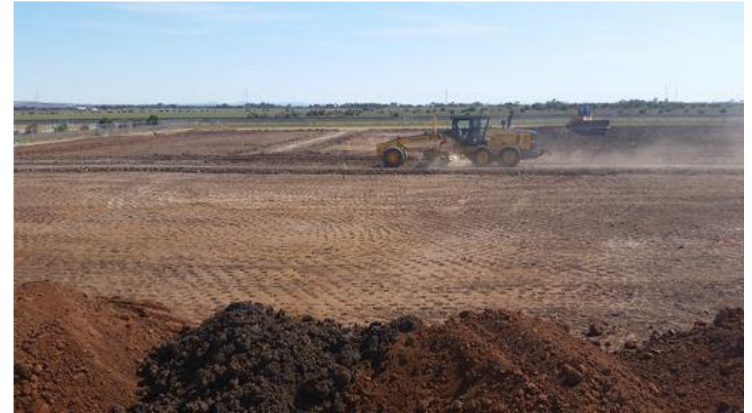
Grader ripping layer 1- G5-G6 (north-east).
