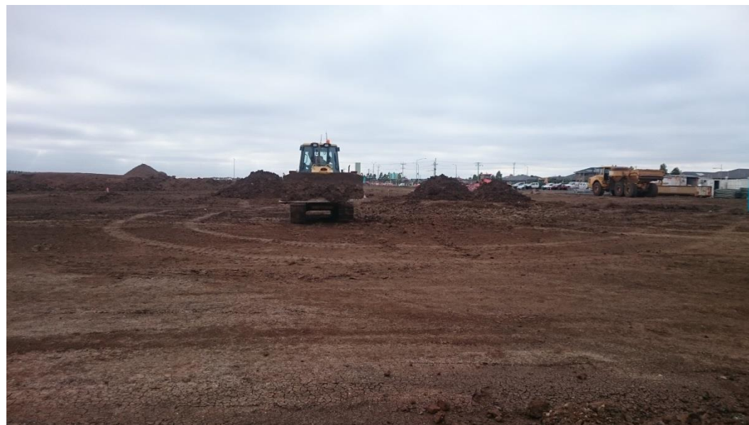
Stage 1: dozer ripping layer 5 prior to placement of layer 6
