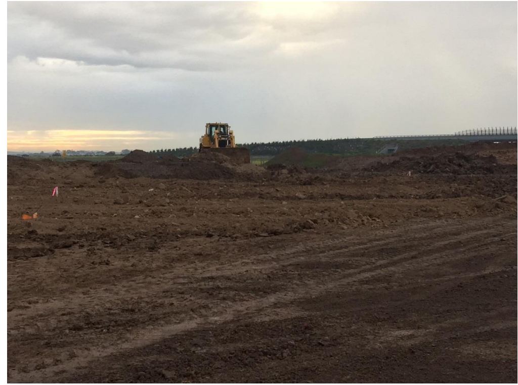
Stage 4: Stockpile being pushed down as fill in grid K5 and L5. Looking NE from grid I5
