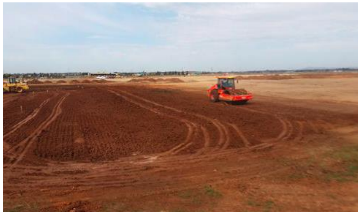
Padfoot Roller compacting layer 1 - column D (east-south-east) and E (west-north-west).
