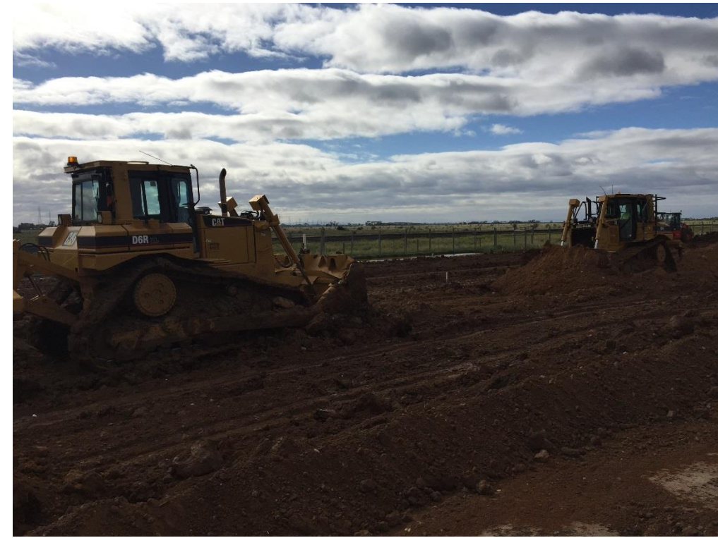
Stage 3: Dozers mixing fill material
