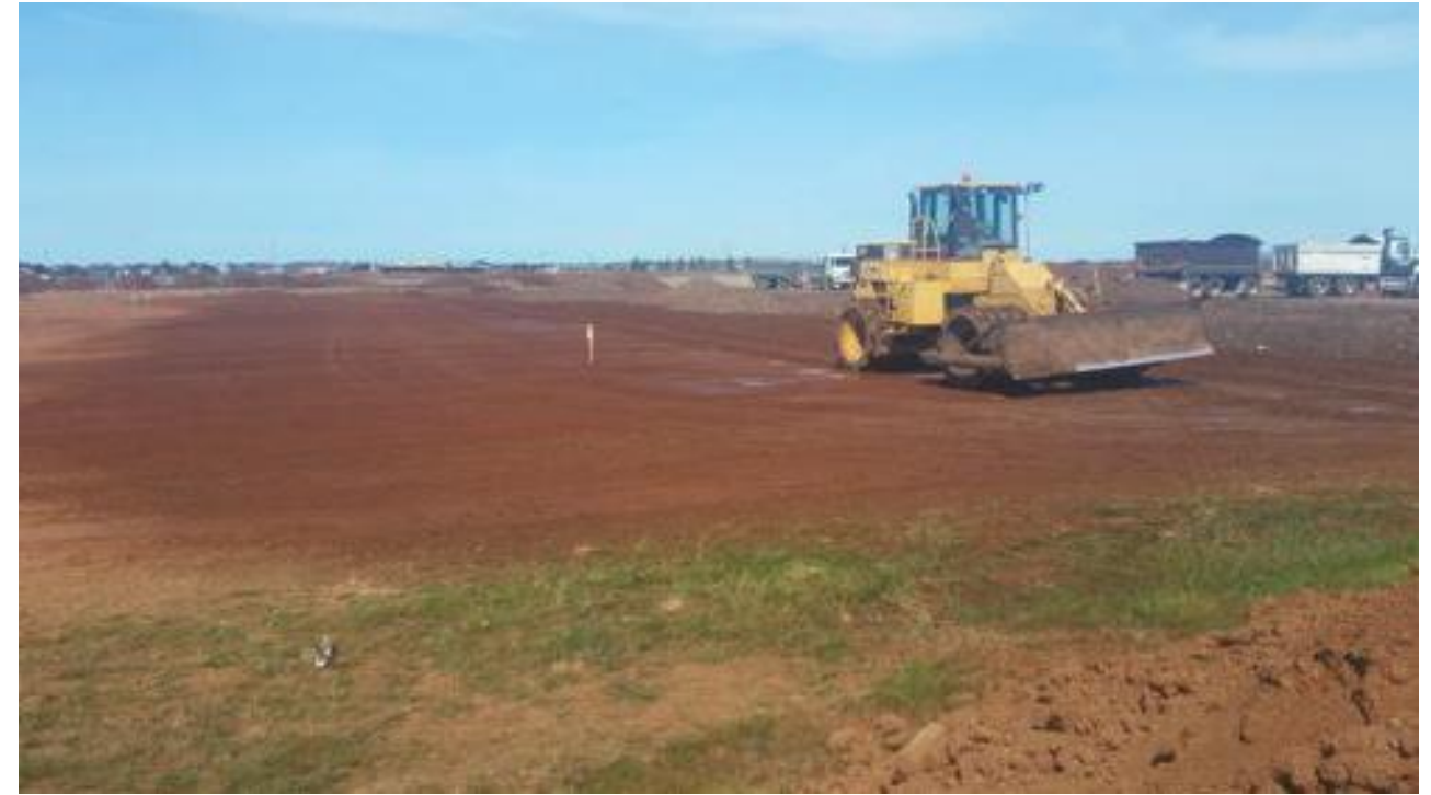
Compactor roughing-up/compacting subgrade prior to layer 1 placement - column D
