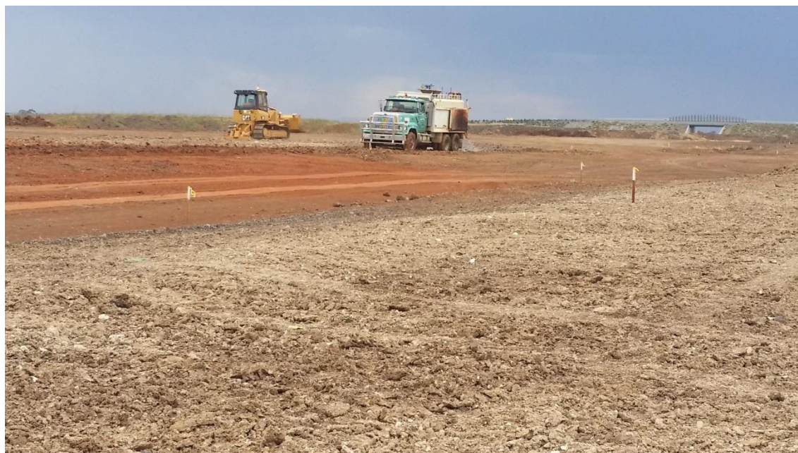
Stage 3: moisture conditioning of scarified layer 3 material in grid B5 (NE), B6 (SE), C5 (N), C6 (S), D5, and D6 (S)
