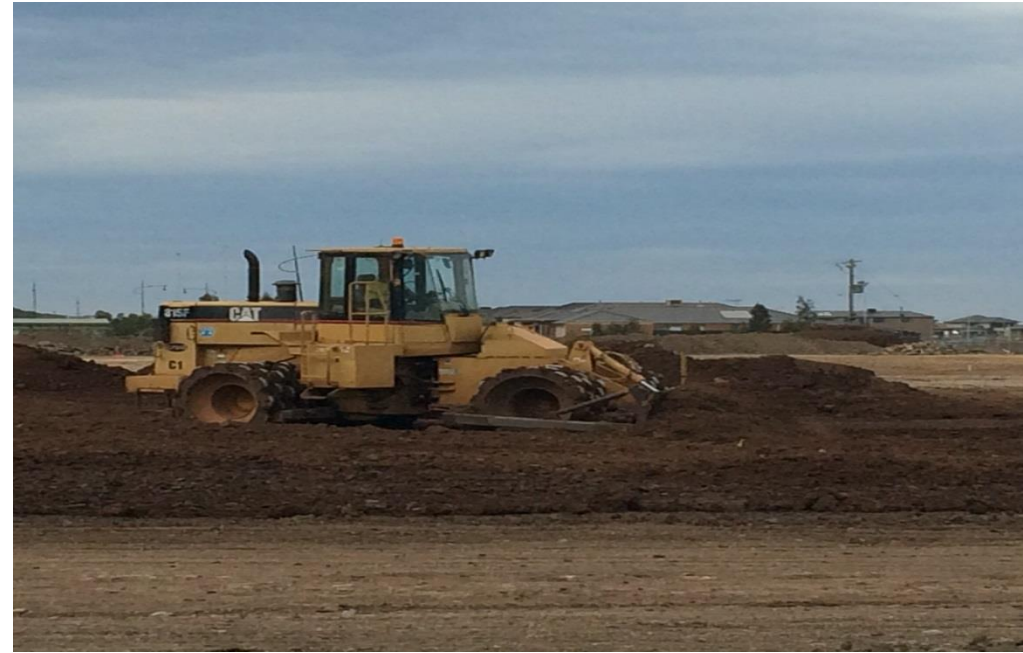
Grader ripping levelling fill from stockpile in layer 1
