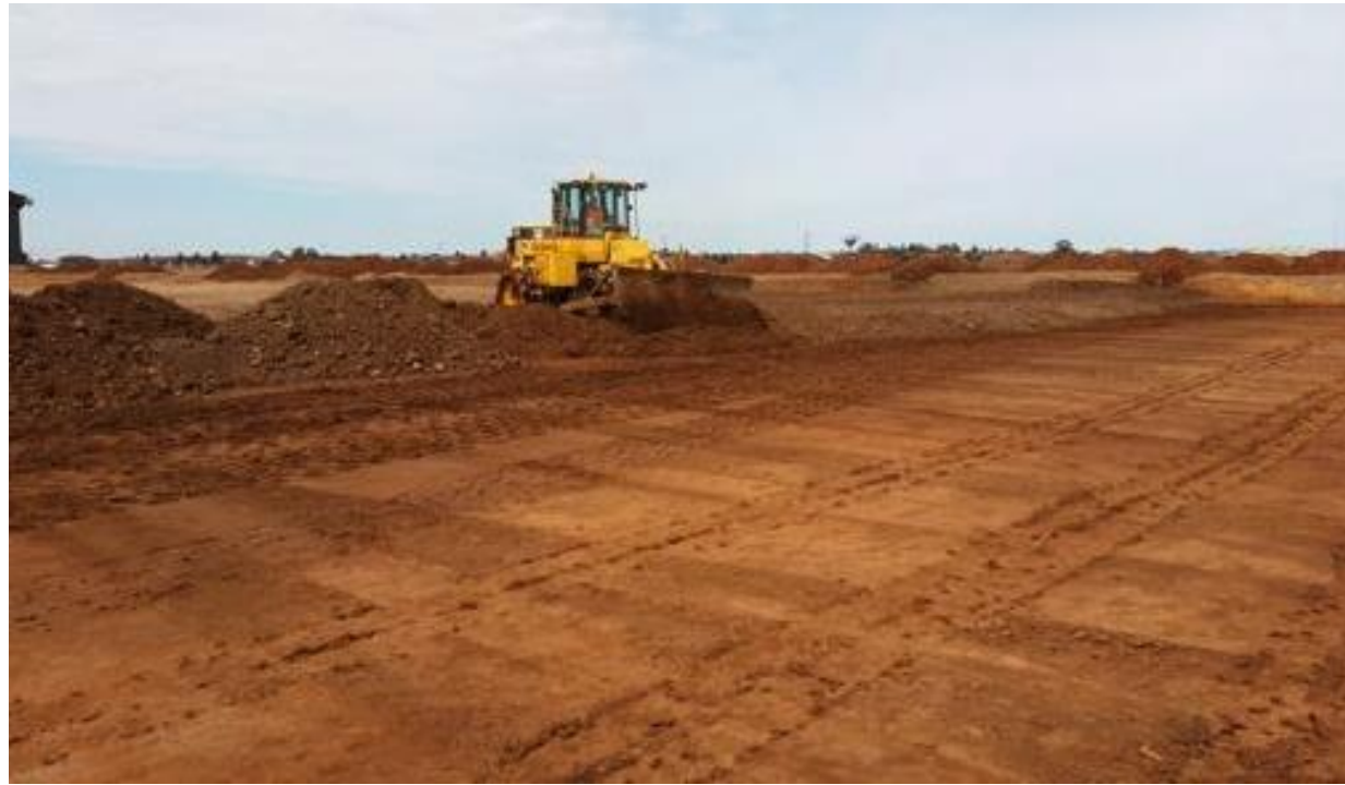
Compactor placing layer 1 - grid column B
