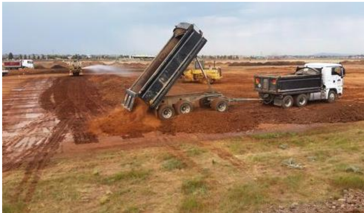
Dump Truck with trailer unloading fill - F6(west-south-west).
