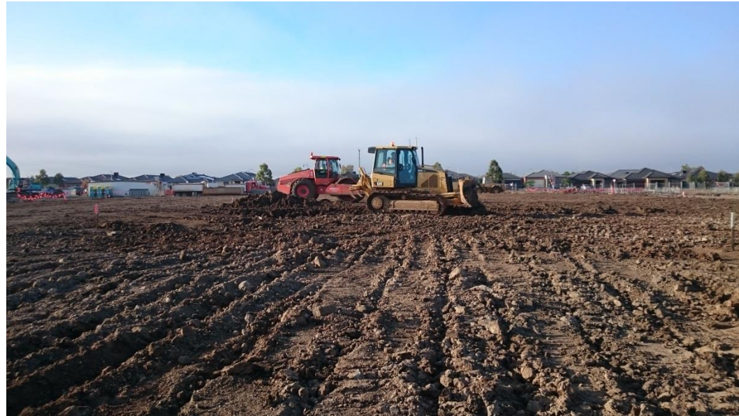
Stage 1: ripped layer 5 being moisture conditioned prior to placement of layer 6 in grid K2
