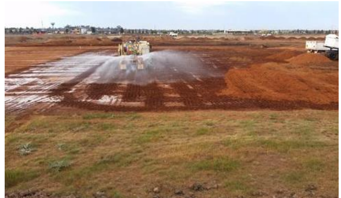
Water Cart moisture conditioning subgrade F5 (west-north-west)/F6(west-south-west).
