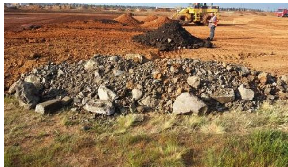
Poorly sorted gravelly/oversize fill from St Albans - E6 (south-south-east)
