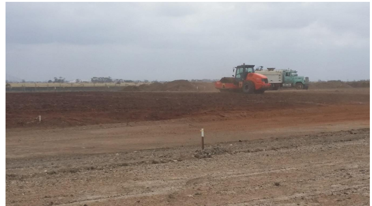
Stage 3: Rolling of worked material in grid B5, B6, C5 (W) and C6 (W).
