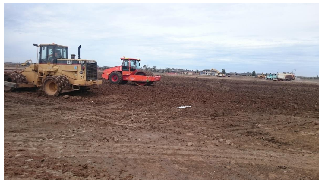
Water cart moisture conditioning Layer 1 in grid G4 (Centre to East) and H4 (West, North-West and South-West)
