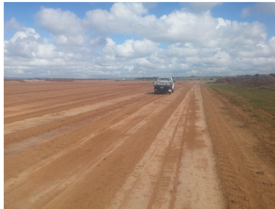
Image 2: Overview of stage 3 (facing west)
