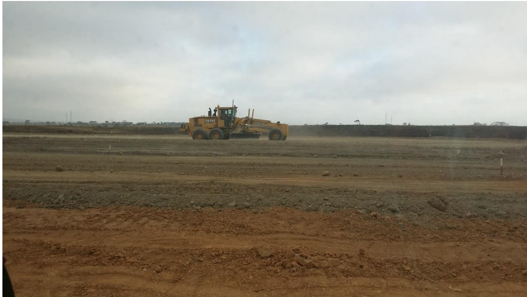
Stage 3: Spreading and grading of material in grid F5 and G5
