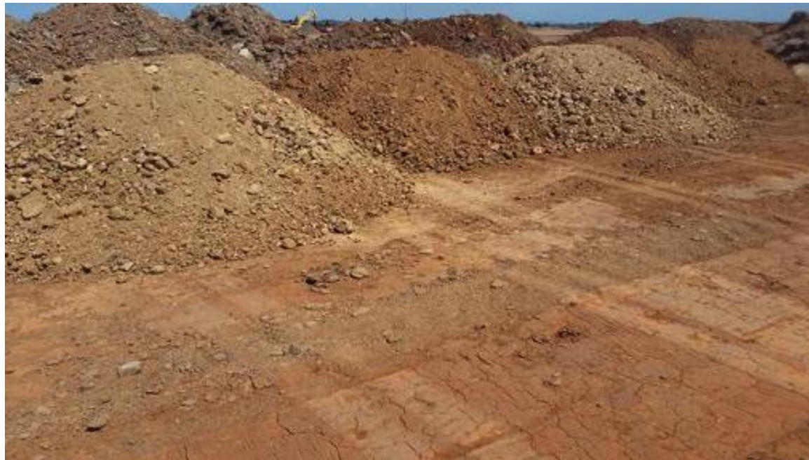
Dry gravelly clay fill (imported from Caroline Springs) - F4 (east-south-east)
