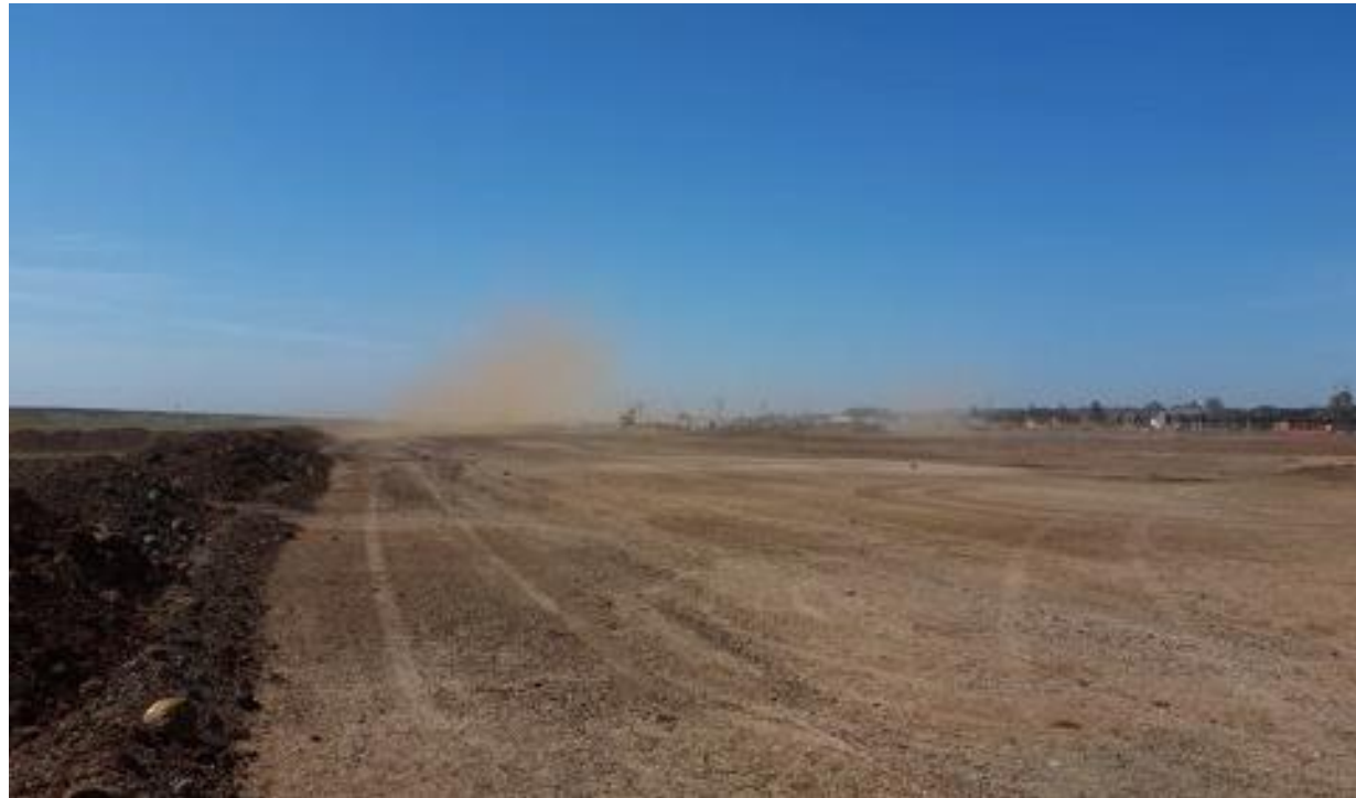
Strong dry winds blowing fill/material off-site
