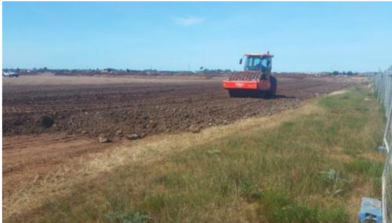
Pad-foot Roller compacting layer 1 – column A
