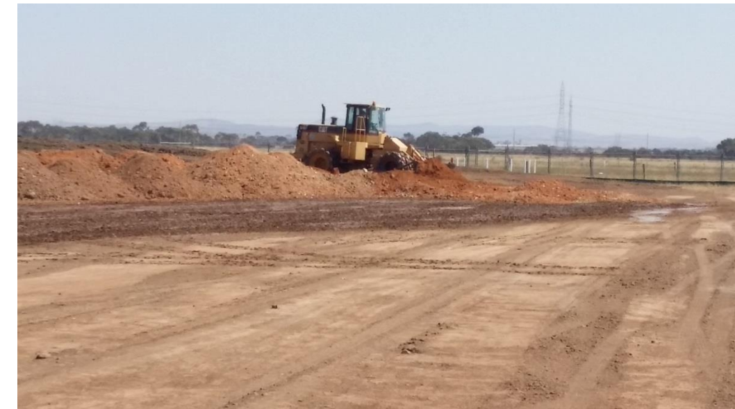
Stage 4: Placing of stockpiled material in grid O3, O4 and O5
