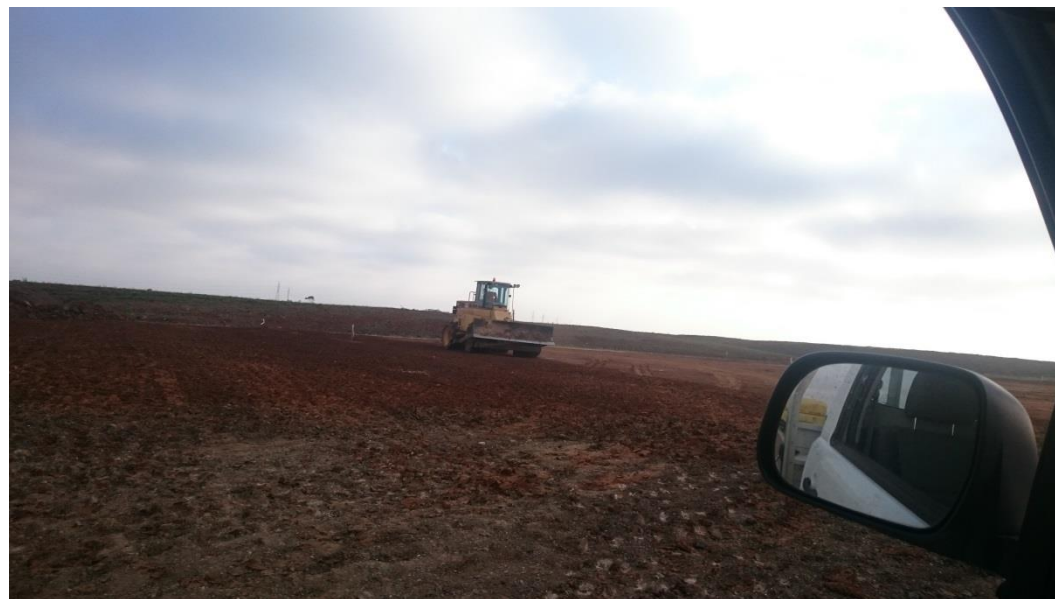
Compactor on layer 2 in grid E5, E6, F5, F6
