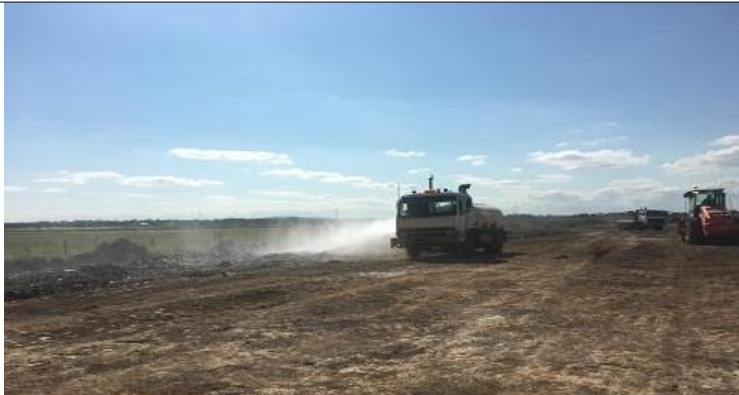
Photo 1 – Looking South-East from H6: Wetting of layer 4 in H6 and layer 2 in G6
