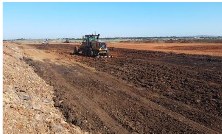
Grader ripping/reworking layer 1 – E4 (north-north-east), F4 (north-north-east), and G4 (west-north-west).
