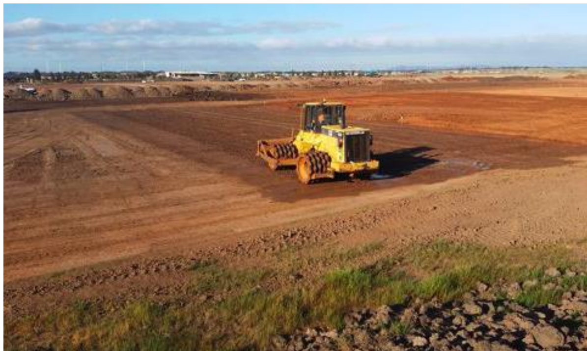
Compactor roughing up/compacting subgrade - G6 (south-west) and G5 (west-north-west).
