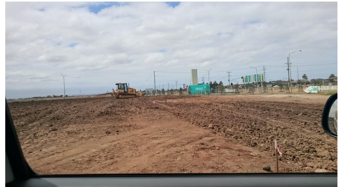
Stage 1: bulldozer ripping layer 5 grid O1 (centre)
