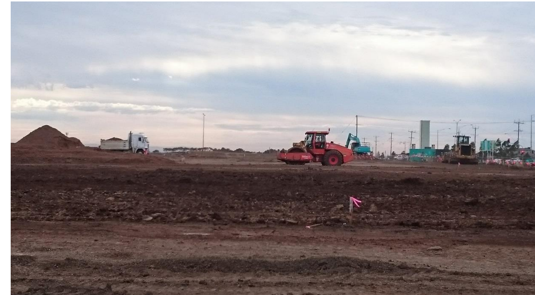
Stage 1: pad foot roller being used on layer 6 in grid L1
