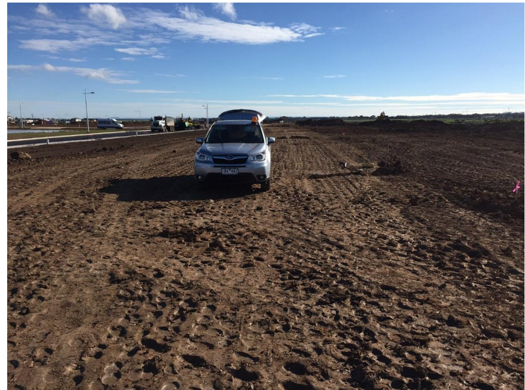
Stage 4: Completed fill placement in grid K5 and L5
