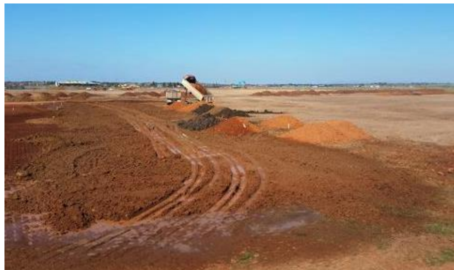
Dump Truck unloading fill – E5 (south-west)
