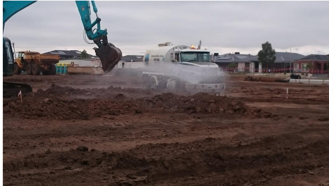
Stage 1: silty clay fill being moisture conditioned prior to placement
