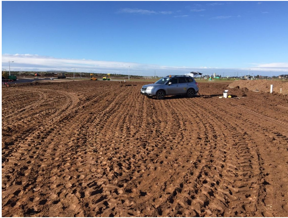
Stage 3: Completed area in grid G4 and H4 . Facing E
