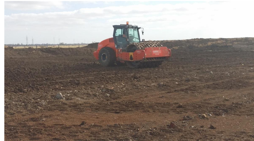
Stage 4: Rolling of layer 2 in grid I5(N), I6(S), J5(NW) and J6(SW)
