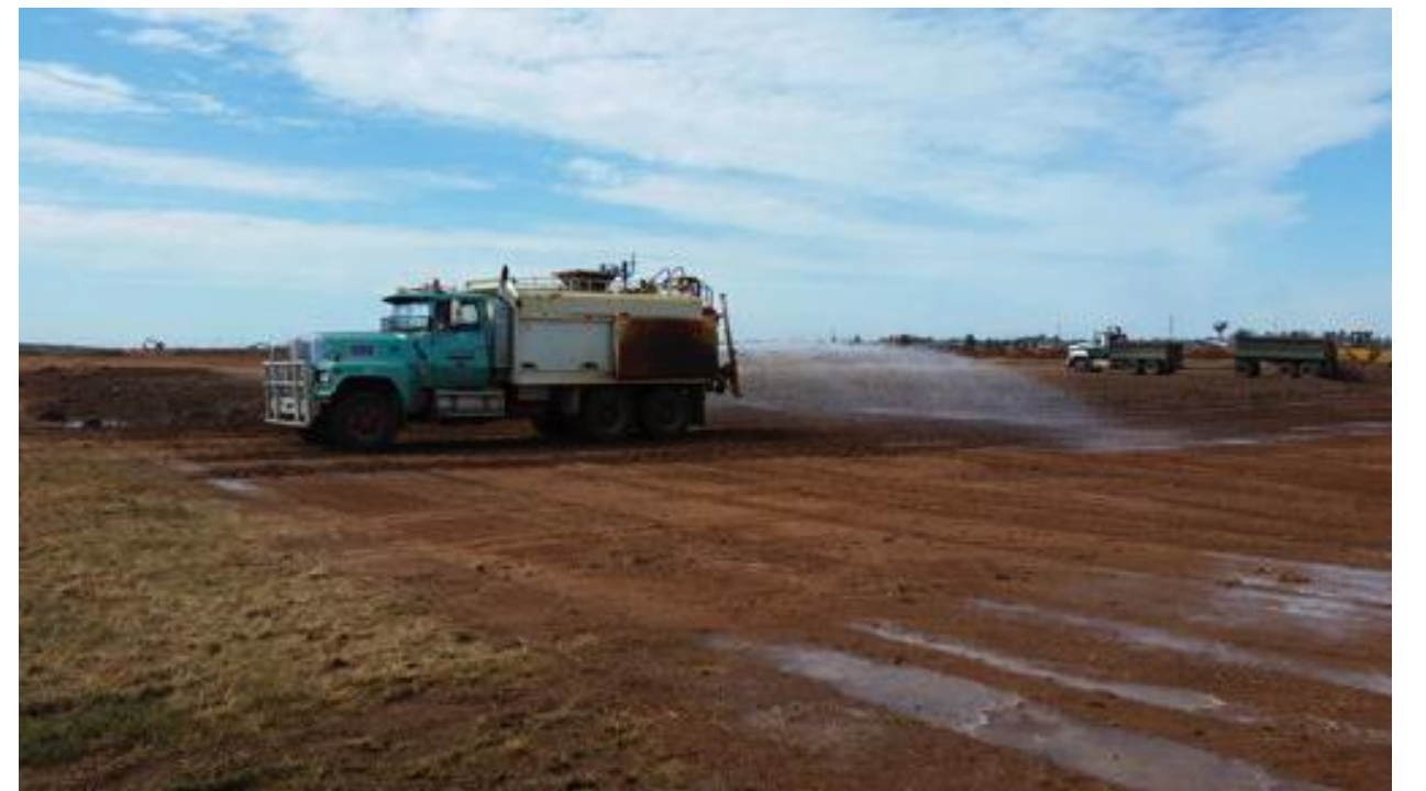
Water truck moisture conditioning subgrade – grid column B
