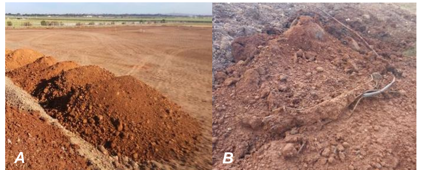
Stockpiled clean fill (A) – C4 (west-north-west), and contaminated fill (B) - E4 (south-east).
