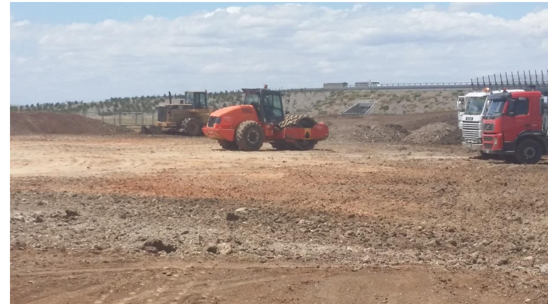
Stage 4: Rolling of layer 1 material in grid L4 (N), L5, M4 (NW) and M5
