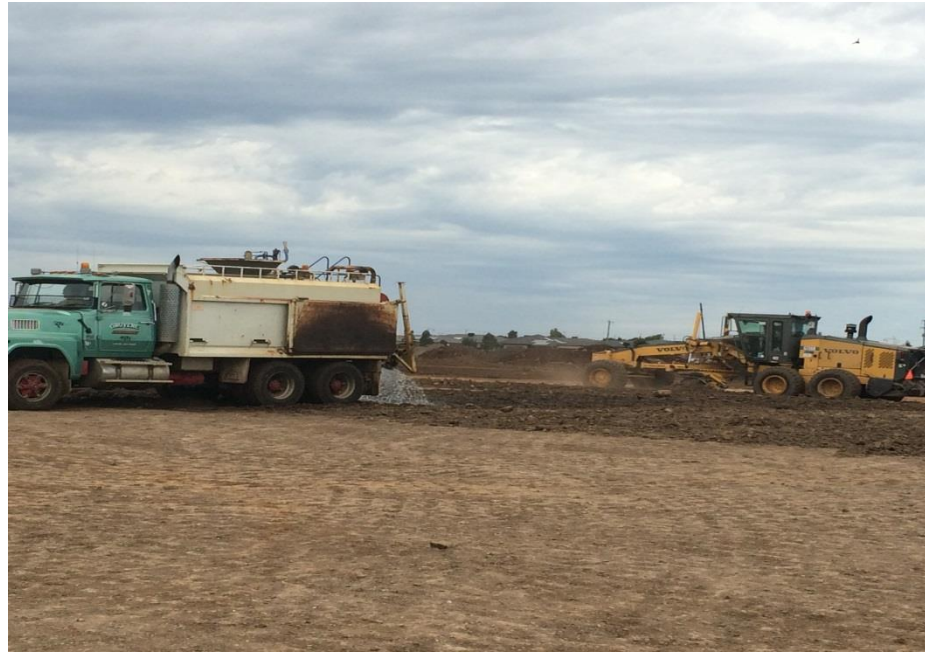
Water cart moisture conditioning Layer 1. and
