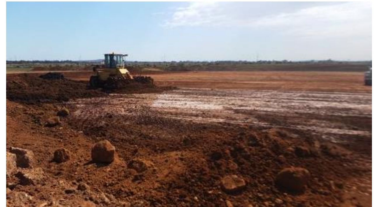
Compactor placing layer 1- E4 (west-north-west).
