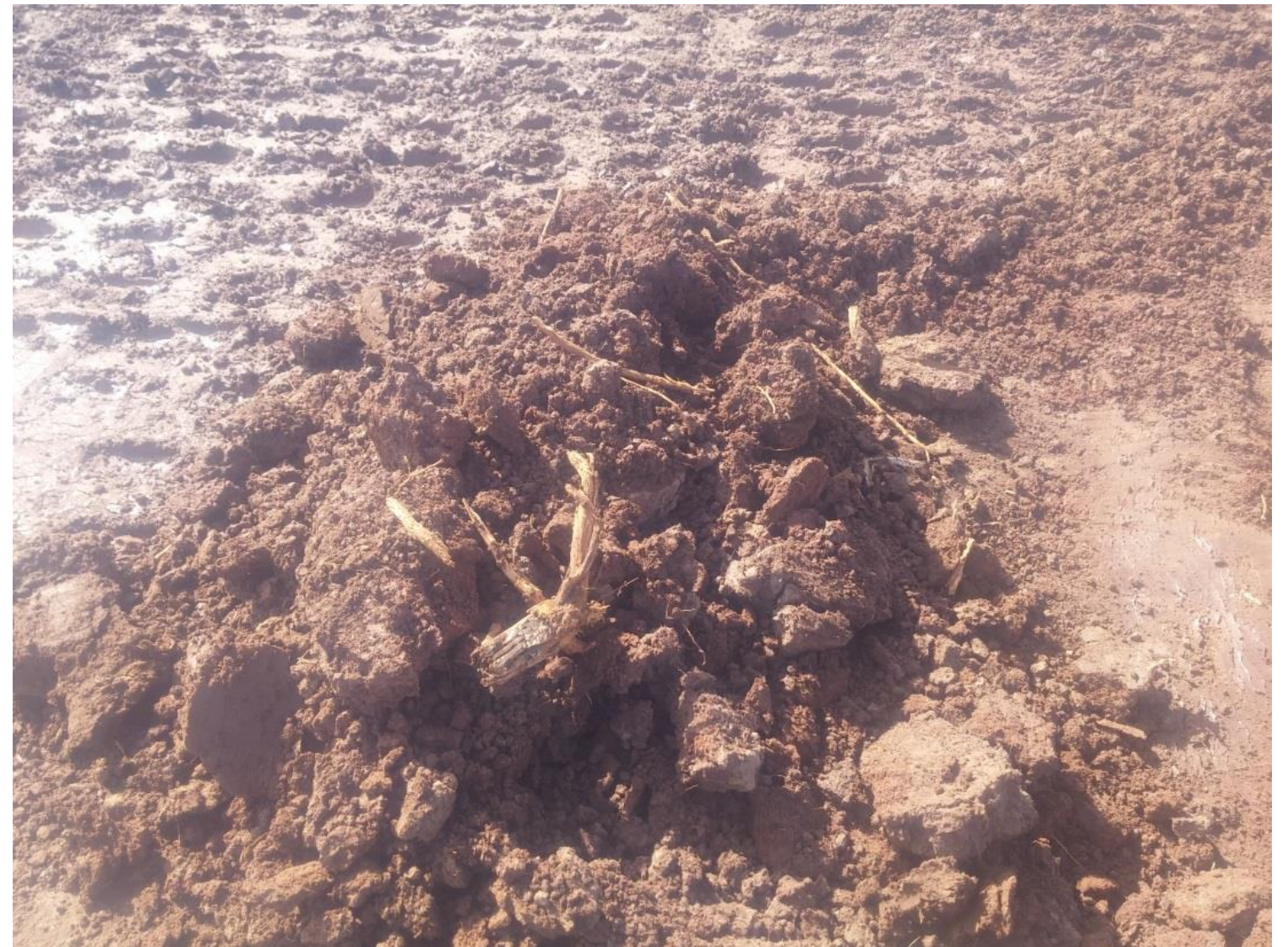
Image 3: Organic roots removed from subgrade with compactor
