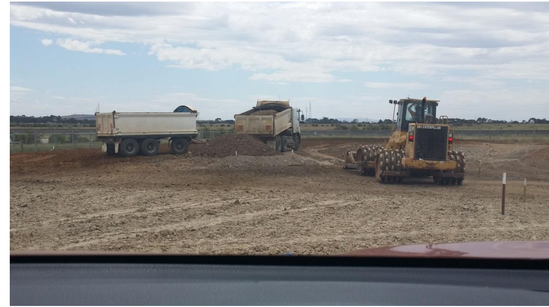
Stage 3: placement of layer 4 in grid A5 and A6
