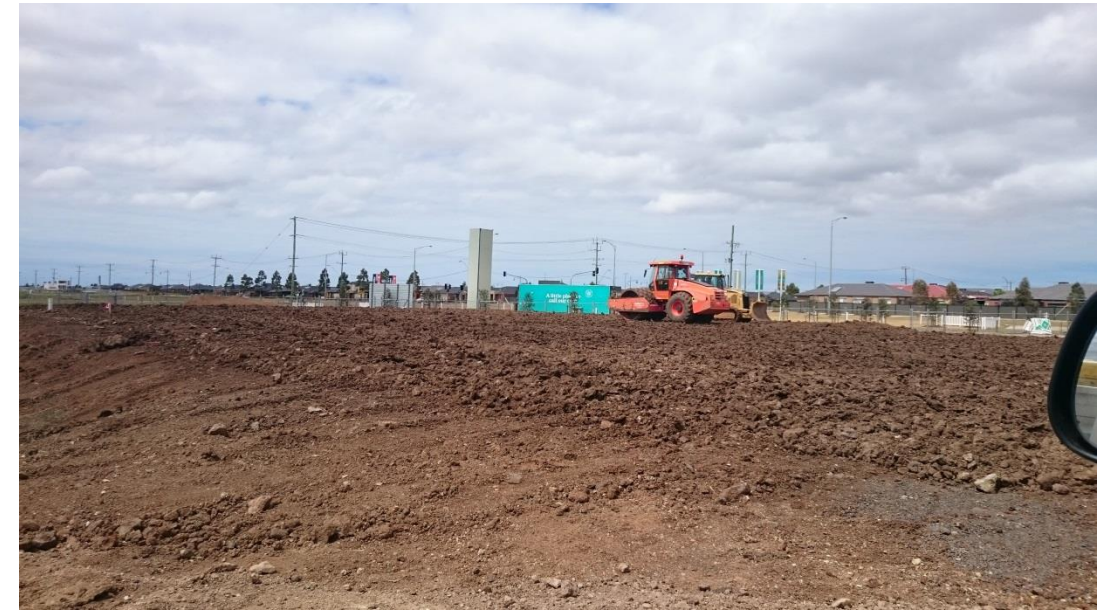
Stage 1: pad foot roller used on layer 7 in grid O1 (North) and O2 (South)
