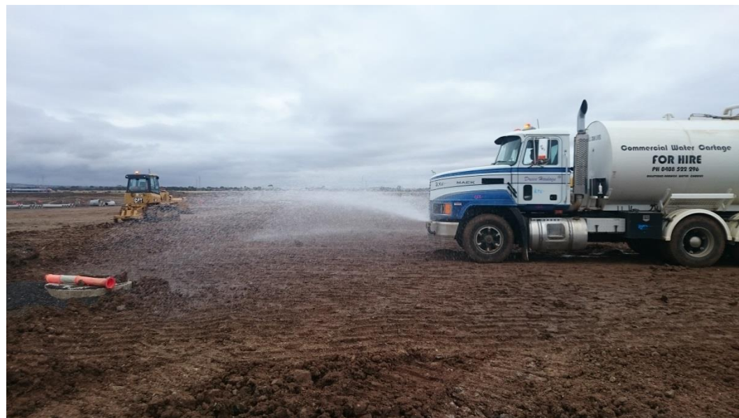
Stage 1: moisture conditioning ripped silty clay material
