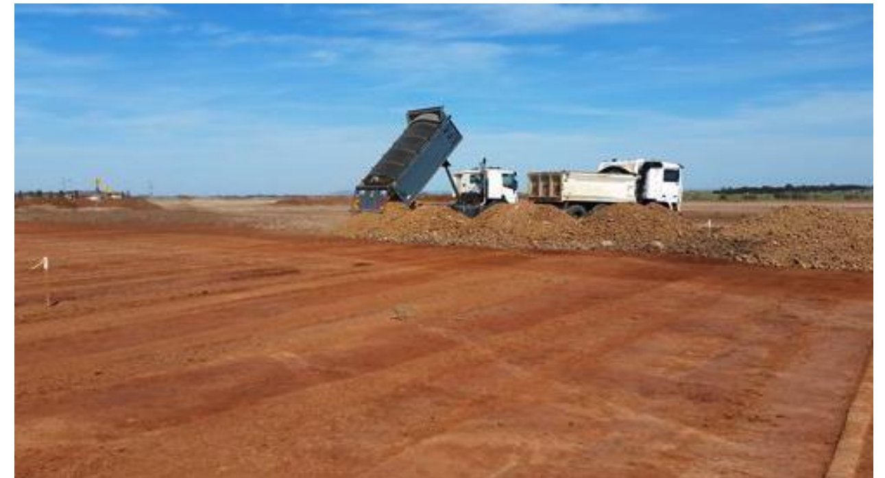
Dump Trucks importing/unloading fill – column D
