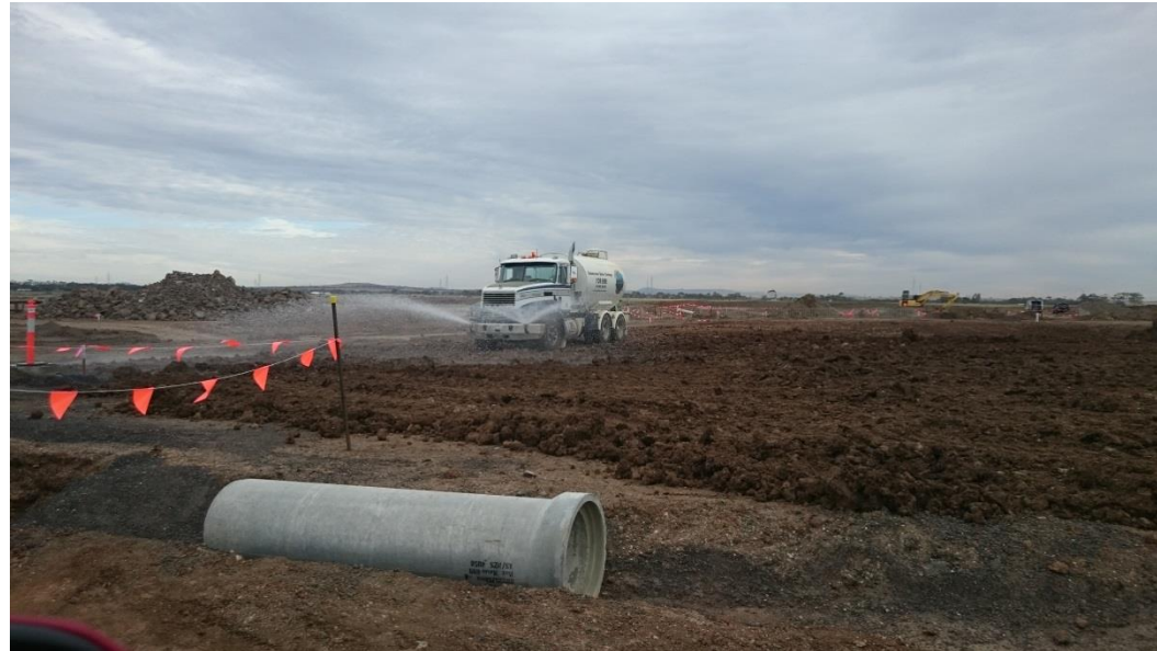
Stage 1: ripped layer 5 being moisture conditioned prior to placement of layer 6
