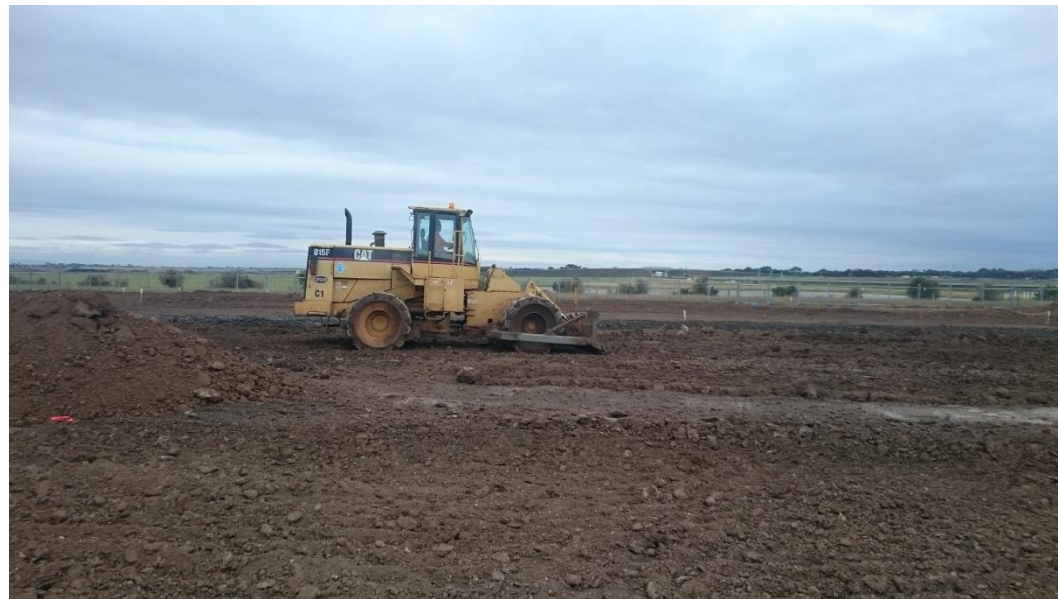
Compactor on Layer 2 in grid B5 and B6
