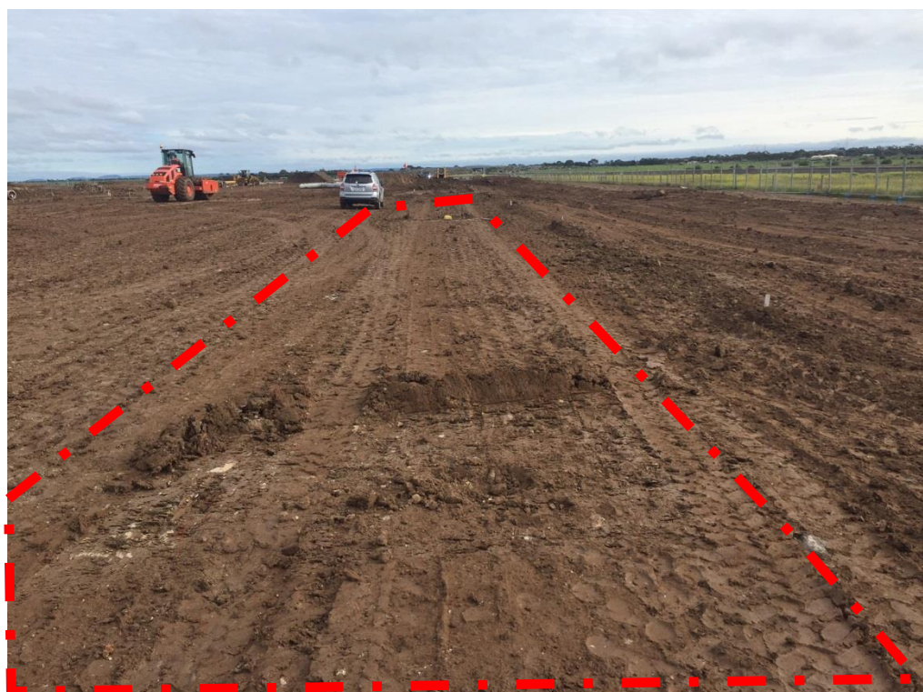
Stage 3: Completed Layer 3 placement in grid section E6,F6 & G6. Facing NW
