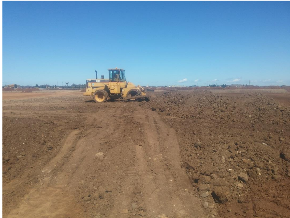
Image 1: Compactor placing layer 1 over grid column C
