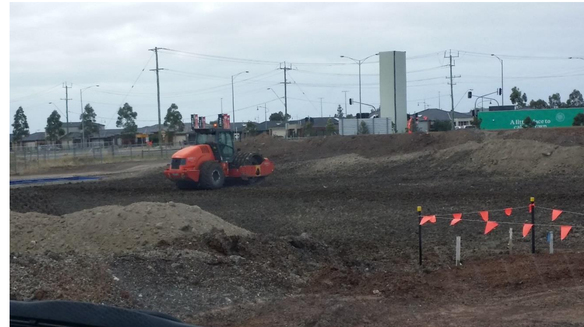
Stage 4: Rolling of placed material in grid N2 (E) and O2
