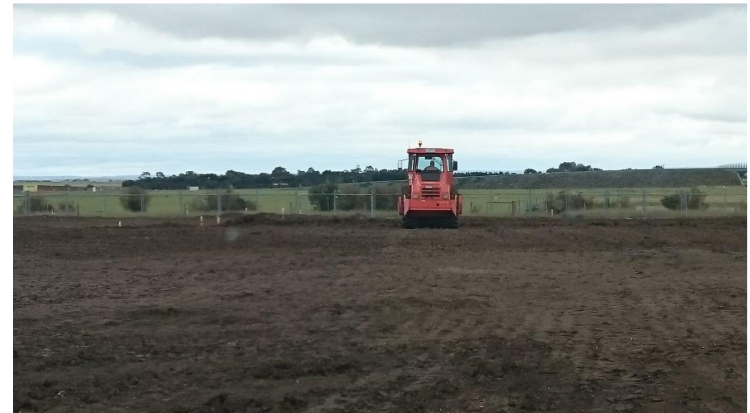
Pad foot roller compacting layer 2 in grid B5 and B6
