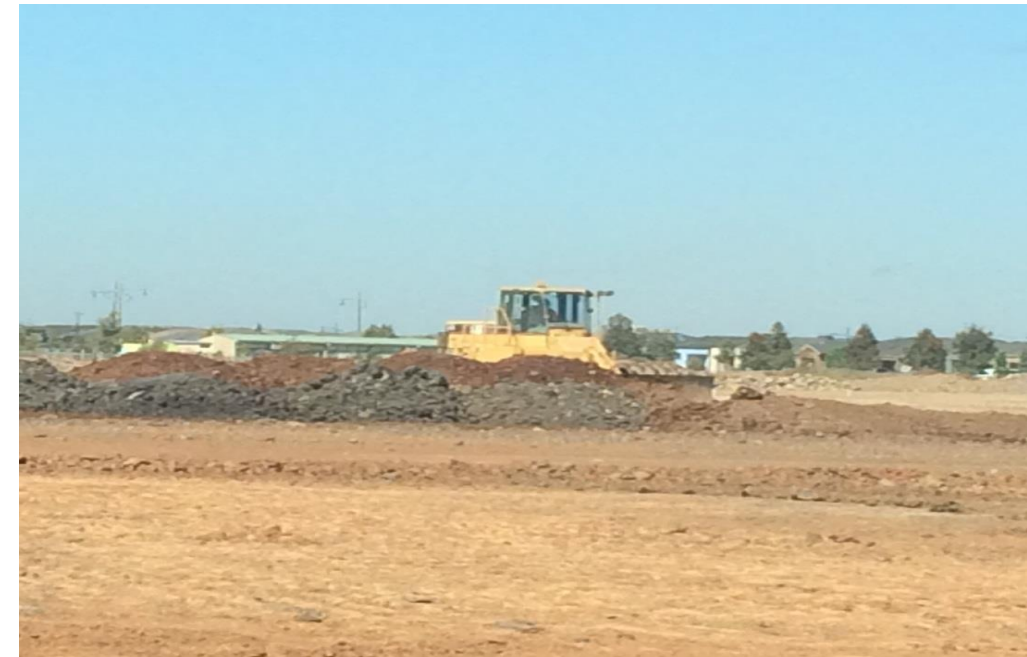
Compactor placing layer 2 grid reference B5-B6
