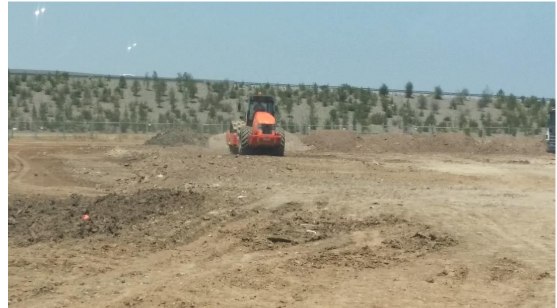
Stage 4: Rolling of placed layer 1 material in grid N4 and N5
