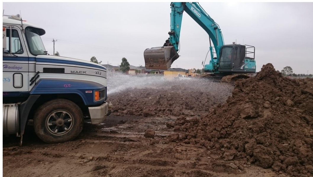
Stage 1: moisture conditioning silty clay material
