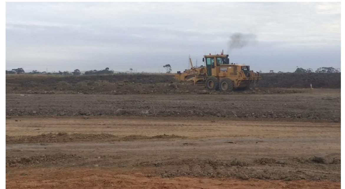
Stage 3: Spreading and grading of stockpiled material in grid F5 and G5
