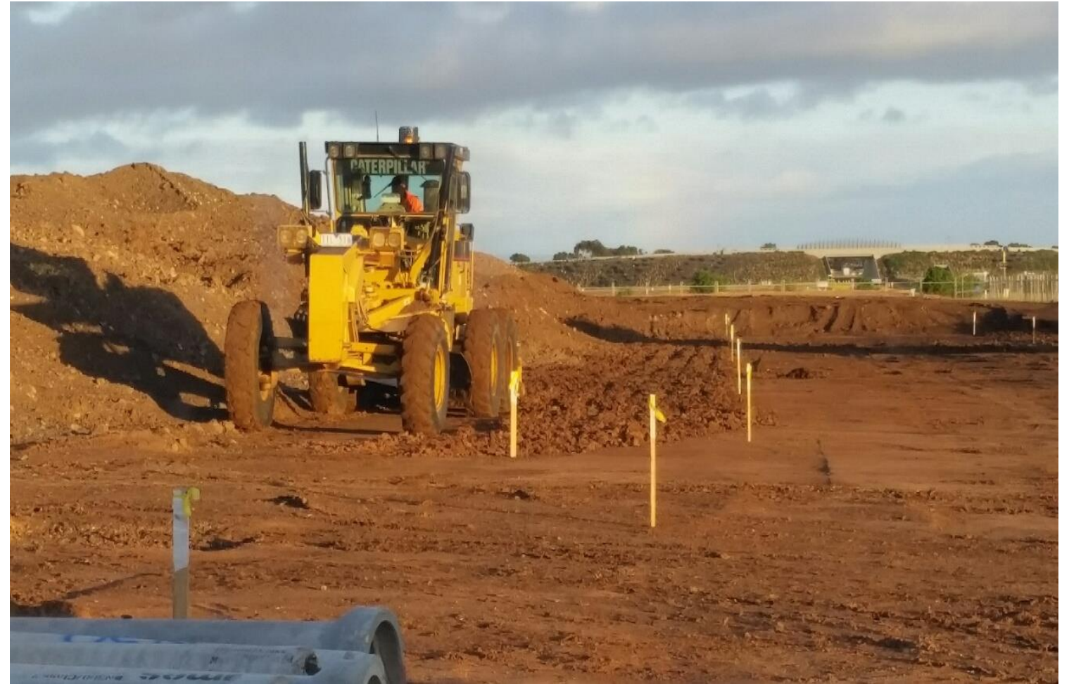
2. Subgrade ripping on grid D6
