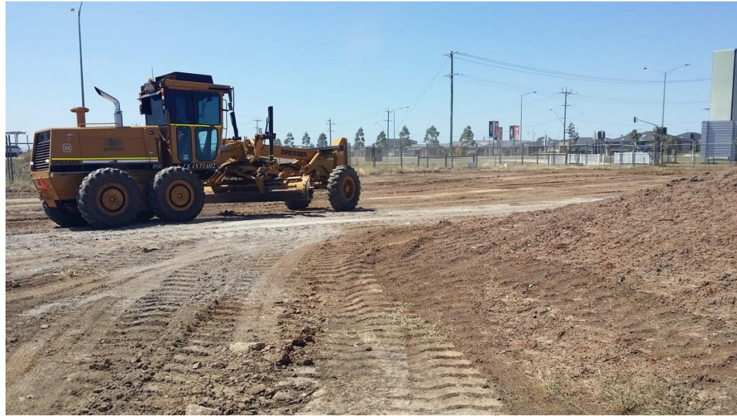
Stage 4: Grader clearing topsoil on subgrade in grid P1 and P2
