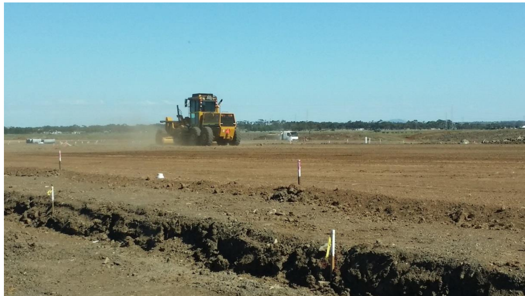
Stage 1: topsoil layer being graded in grid K3
