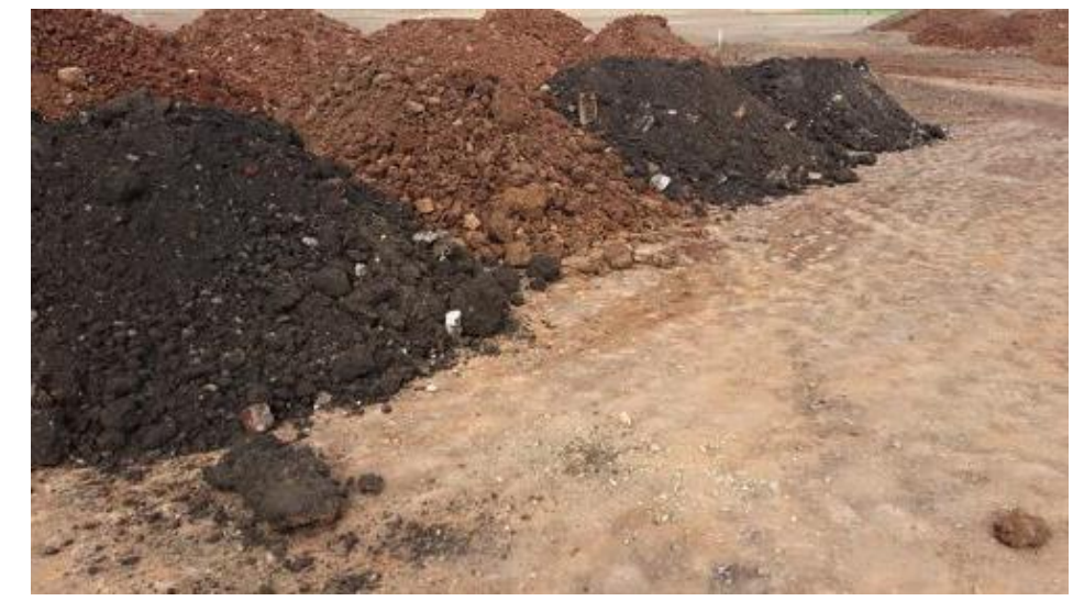
St Albans fill stockpiled for quality control D4 (north)
