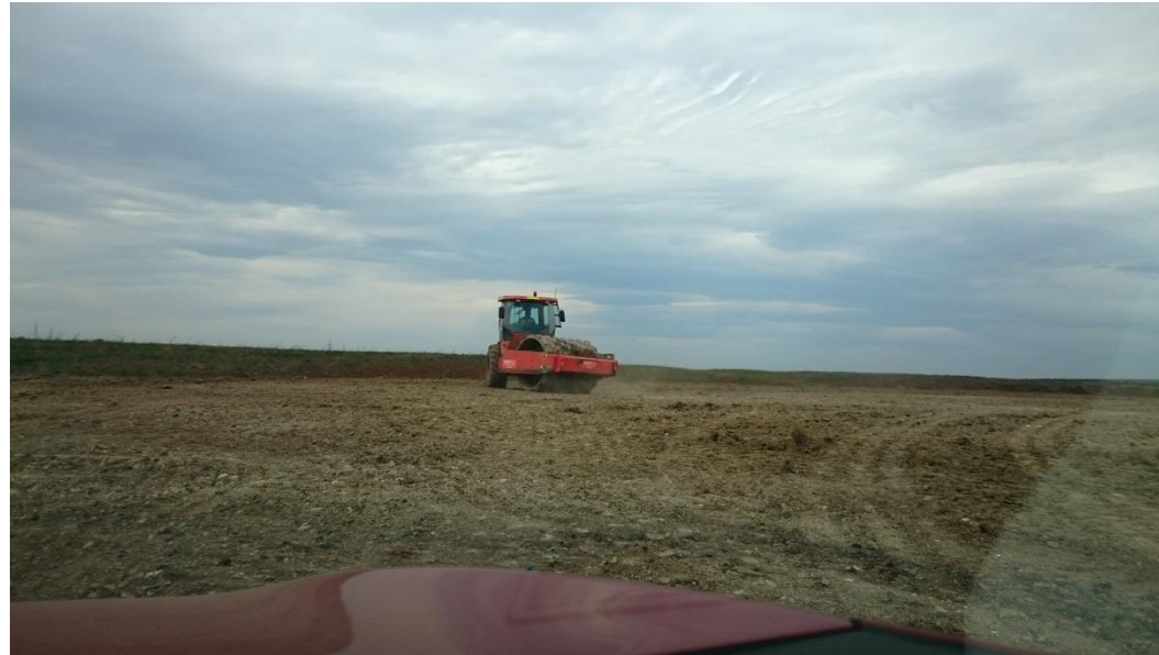
Stage 3: pad foot roller on layer 3 after being re-worked in grid E5, E6, F5, F6, G5 (W) and G6 (W)
