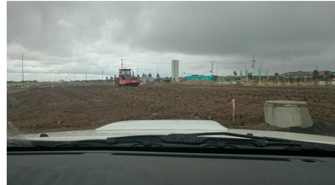
Stage 1: Compactor used on layer 7 in grid O1 (North) and O2 (North) to compact on-site fill that was moisture conditioned
