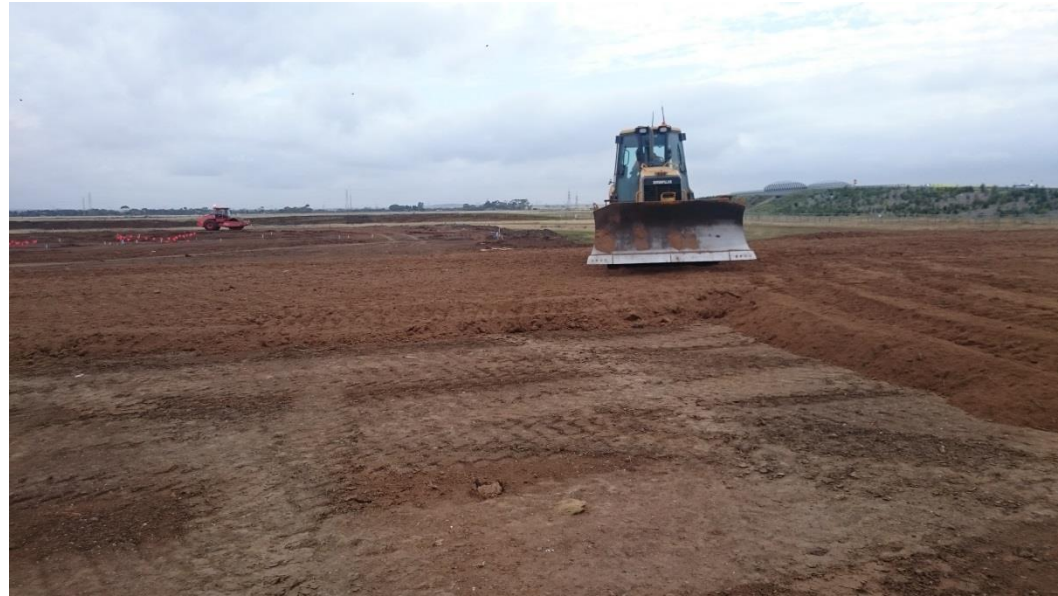
Stage 1: placement of topsoil in in grid O1 and O2
