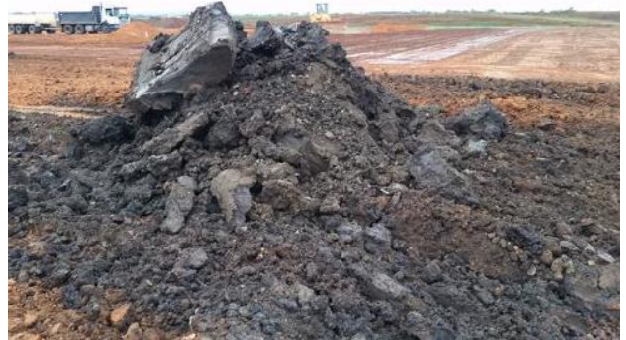
St Albans clay fill - F4 (north-east).
