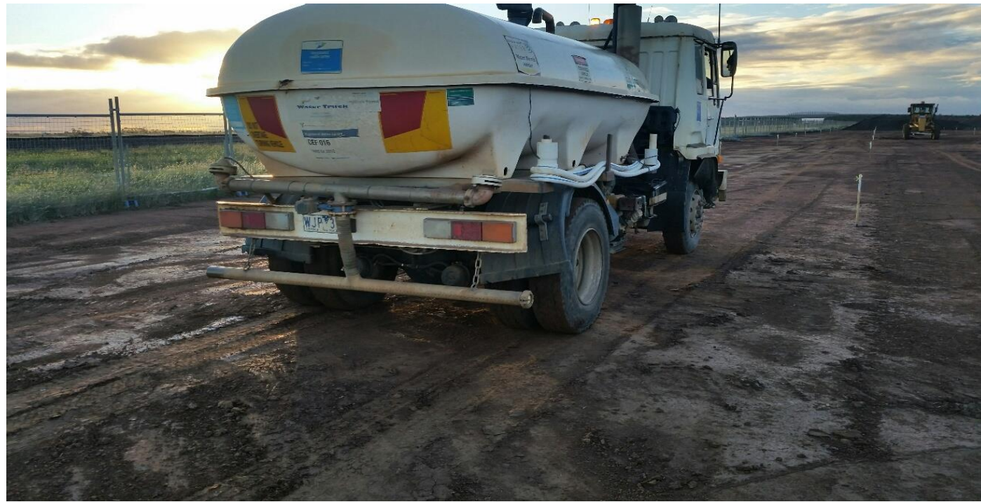
1. Proof roll has been done with water cart
