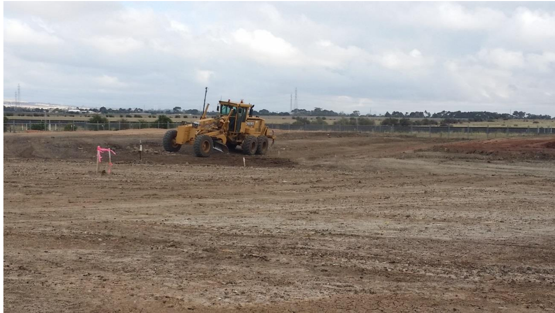
Stage 3: Building up of material in roadways.
