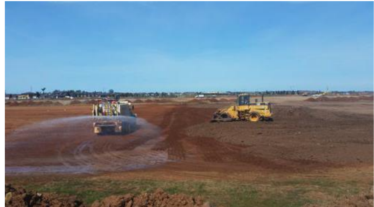
Water Cart moisture conditioning subgrade prior to/during layer 1 placement – column D
