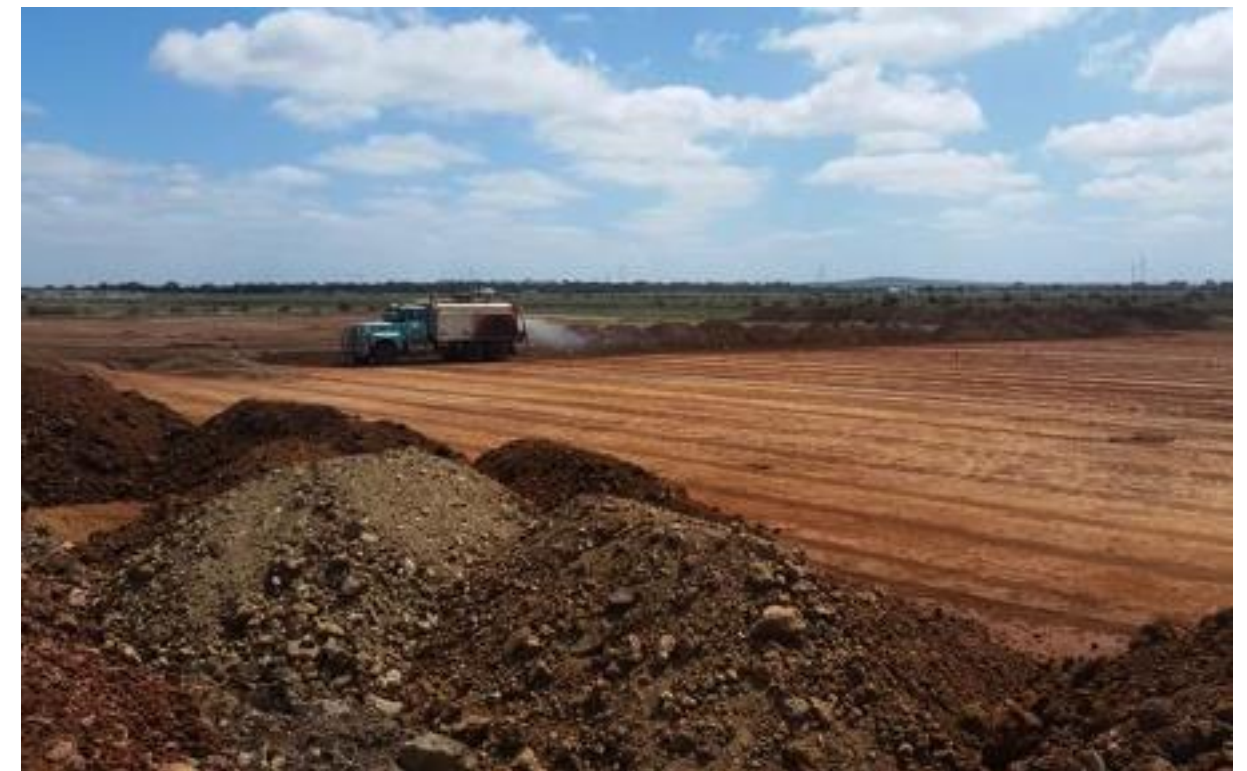
Water Cart moisture conditioning stockpiled fill - D5 (north-east)
