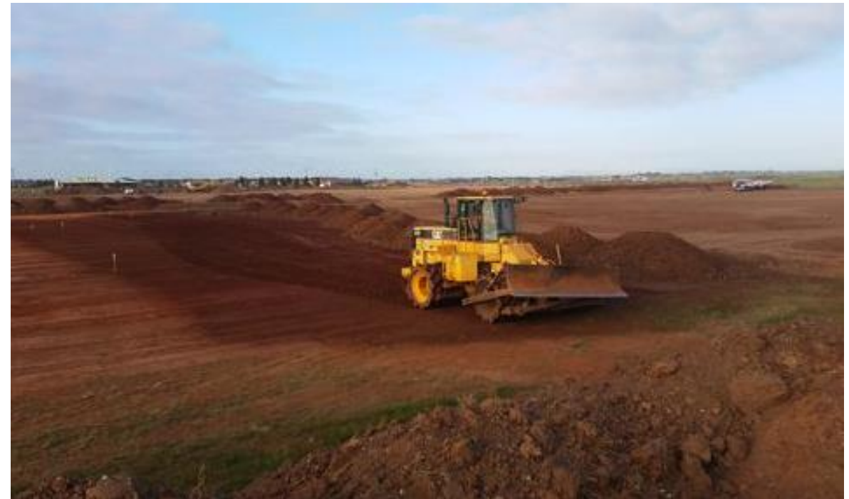
Compactor roughing-up/compacting subgrade - column D (east-south-east) and E (west-north-west).
