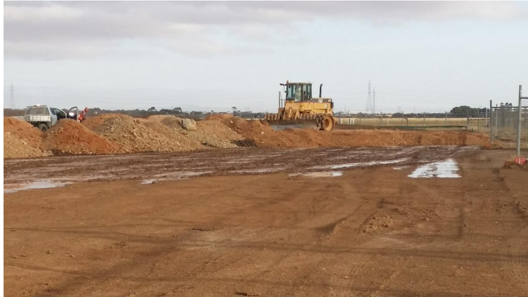
Stage 4: Placing of layer 1 material in grid N3 (E), O3, O4 (E), and O5 (E)
