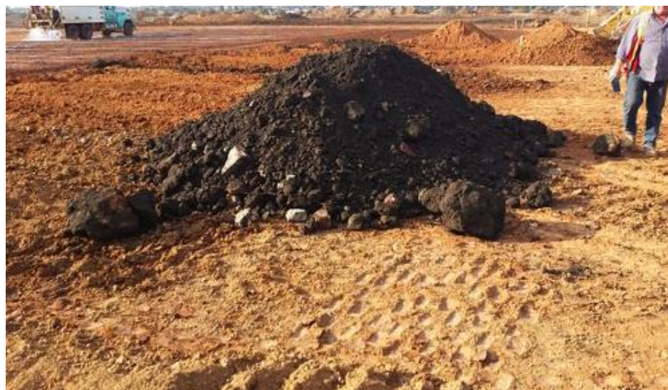
St Albans gravelly clay fill with some oversize - E6 (south-south-east)
