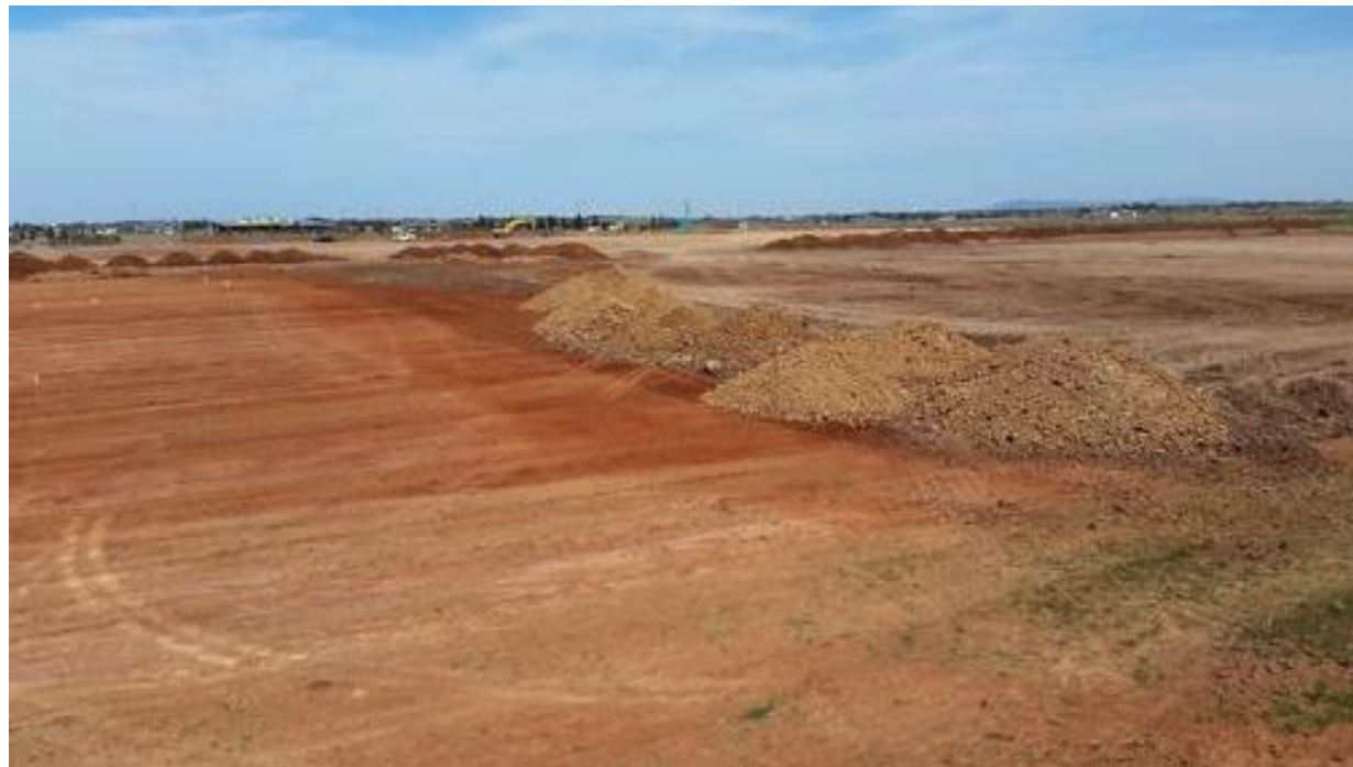
Stockpiled fill – column D
