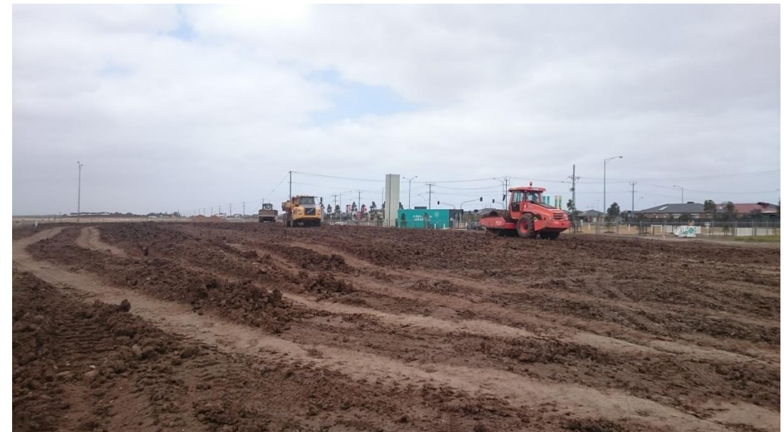
Stage 1: bulldozer placing layer 7 in grid O1 (North) and O2 (South)
