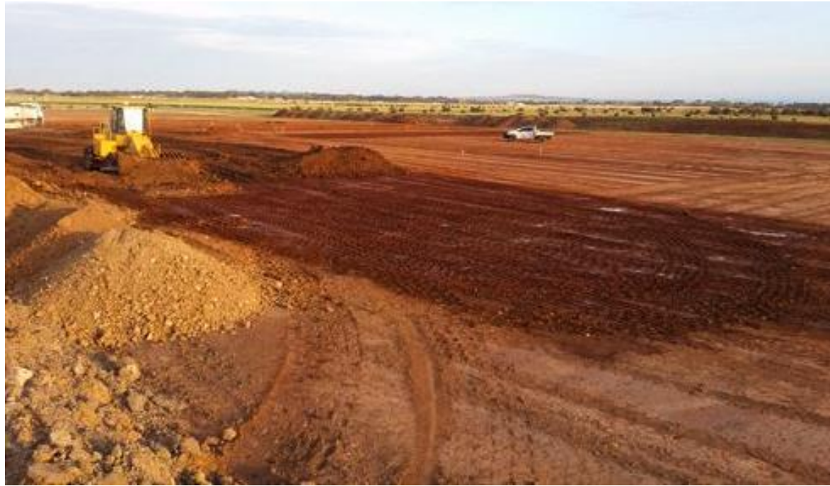
Compactor placing layer 1 – F4 (north)
