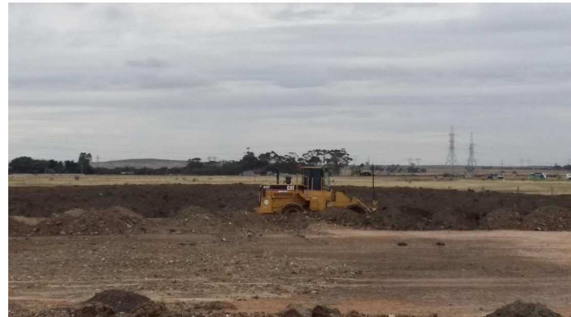
Stage 4: Placement of layer 1 in grid K6 (S), L6 (S), M6 (S), N6 (S) and O6 (S).
