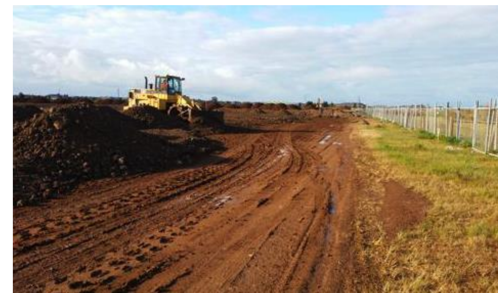
Compactor placing layer 1 – Column A
