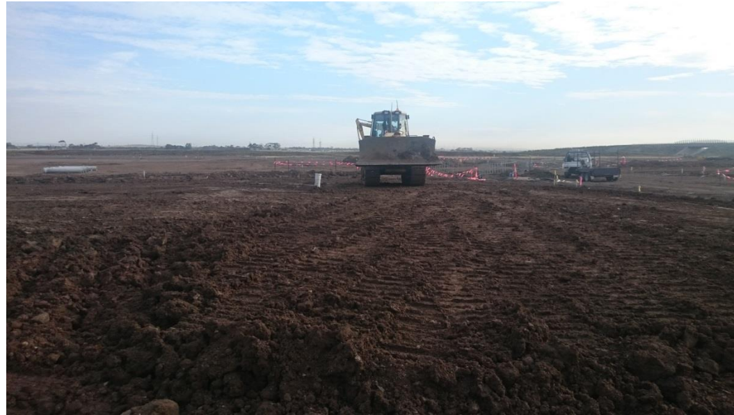
Stage 1: placement of layer 6 in grid J2
