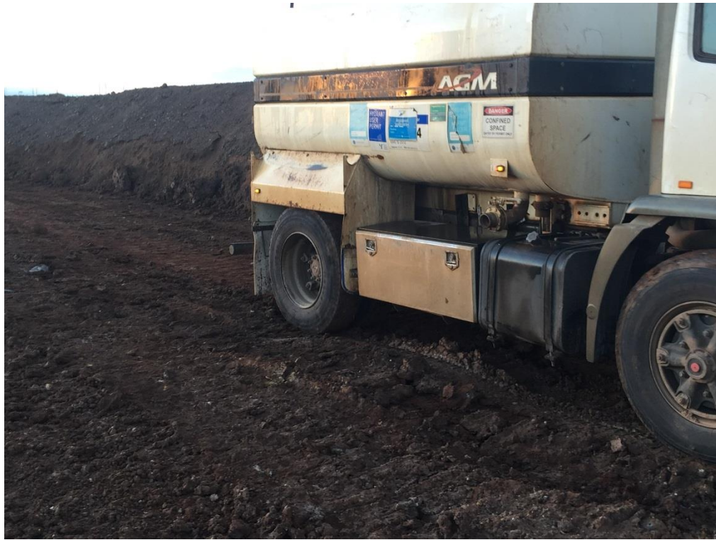
Stage 3: Proof rolling subgrade area within previous stockpile location. Facing E
