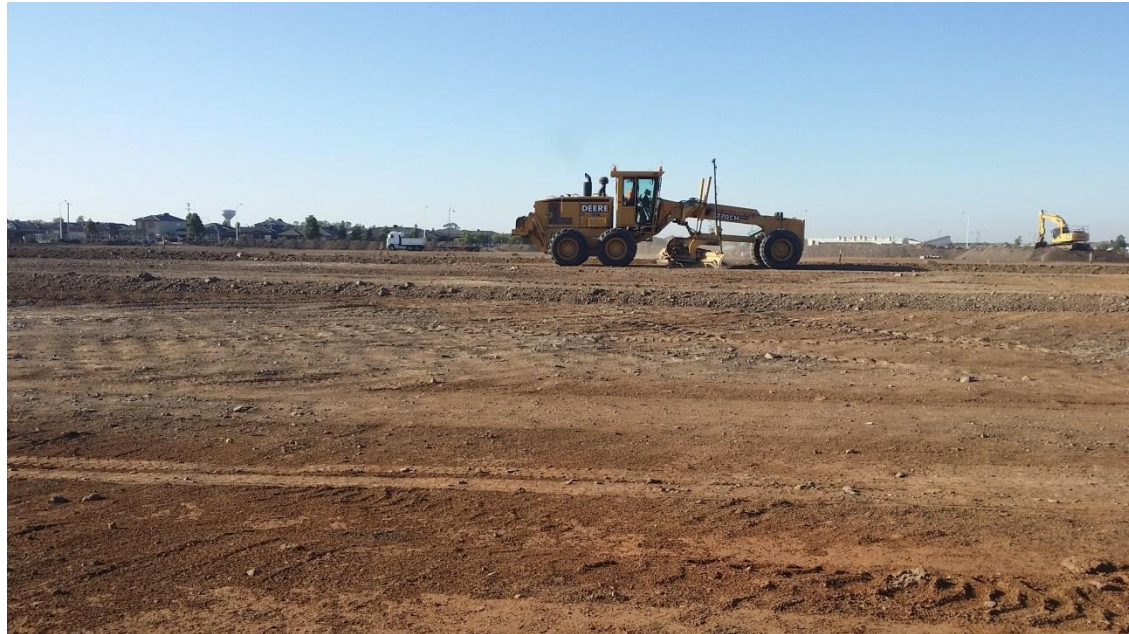
Stage 3: Spreading and grading of material in grid D4 (N), E4, F4 and G4
