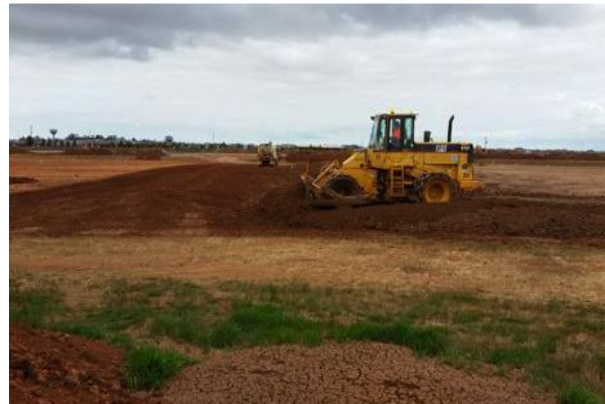
Compactor placing layer 1 - Column C
