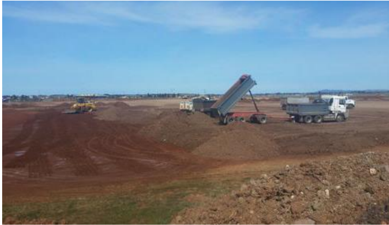
Dump trucks unloading fill – column D
