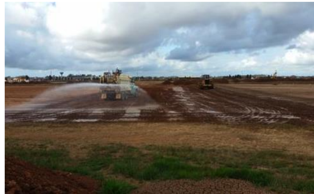
Water truck moisture conditioning subgrade – Column C
