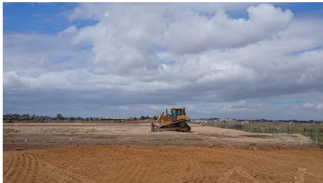
Stage 3: topsoil layer being placed in grid A4, B4 and C4
