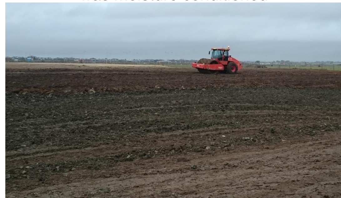
Stage 1: Compactor used on layer 7 in grid O1 (North) and O2 (North) to compact on-site fill that was moisture conditioned
