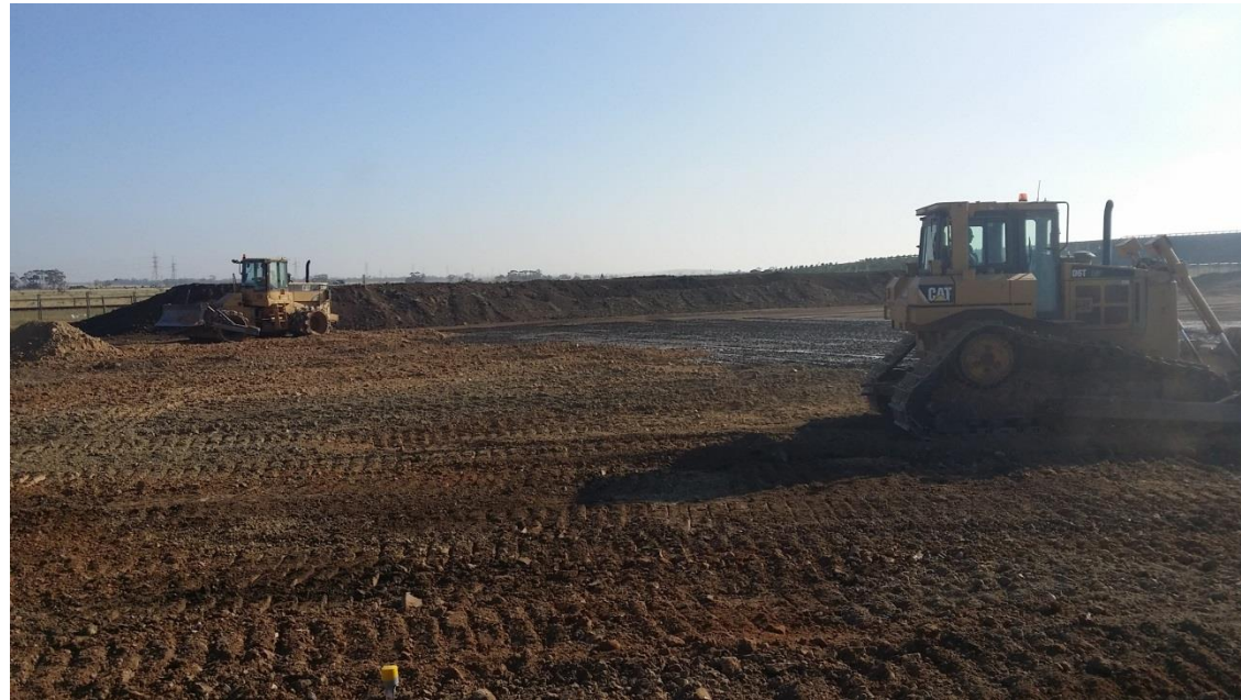
Stage 4: Placement and compaction of layer 1 material by CAT compactor in grid J5, J6 (S), K5 and K6 (S)
