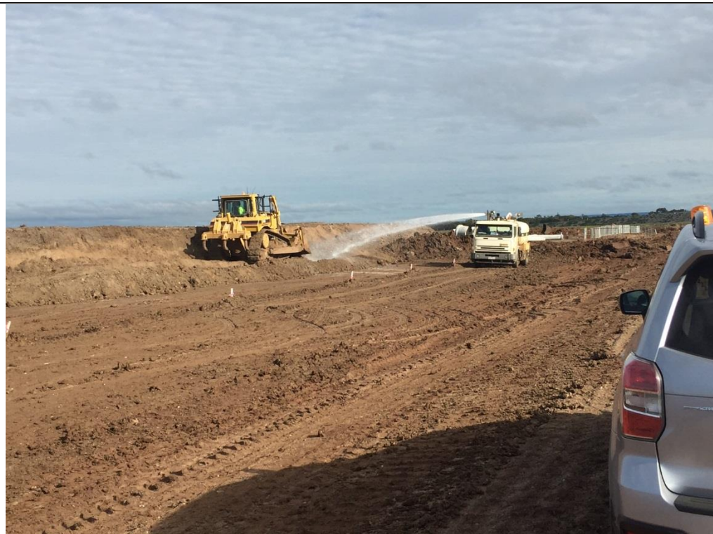
Stage 3: Moisture conditioning fill stockpile while being pushed down
