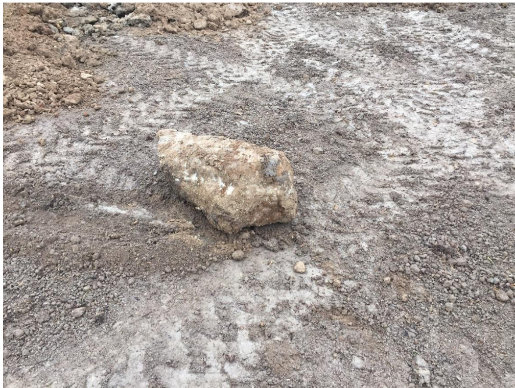
Stage 4: Boulders was removed during fill placement
