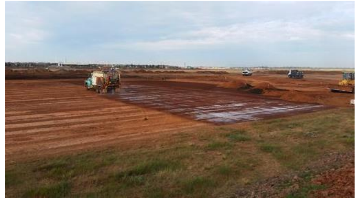
Water Cart moisture conditioning subgrade - E5 (east)/E6 (south-south-east).
