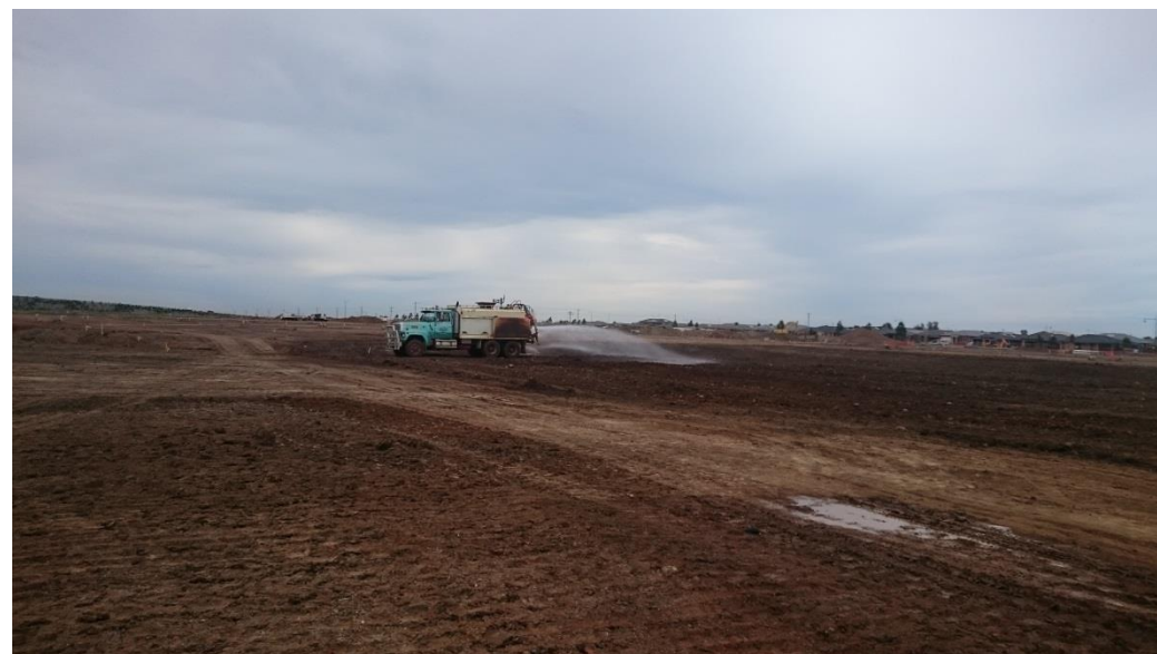
Water cart moisture conditioning Layer 1 in grid G4 (Centre to East) and H4 (West, North-West and South-West)
