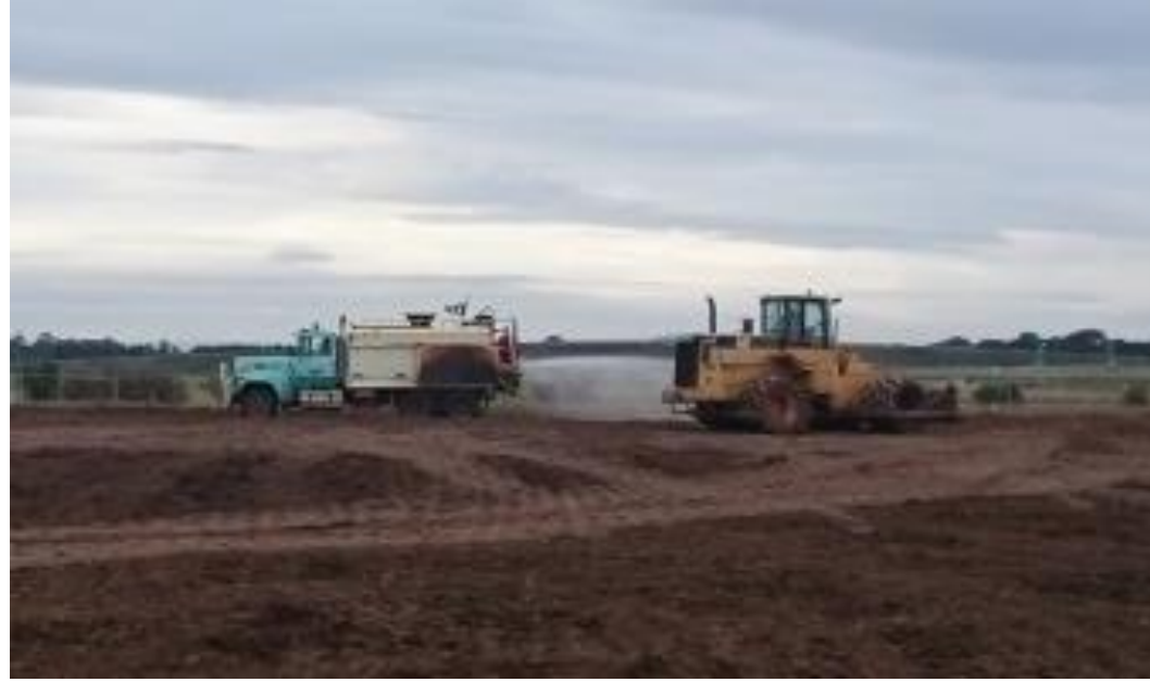
Water cart moisture conditioning layer 2 in grid B5 and B6
