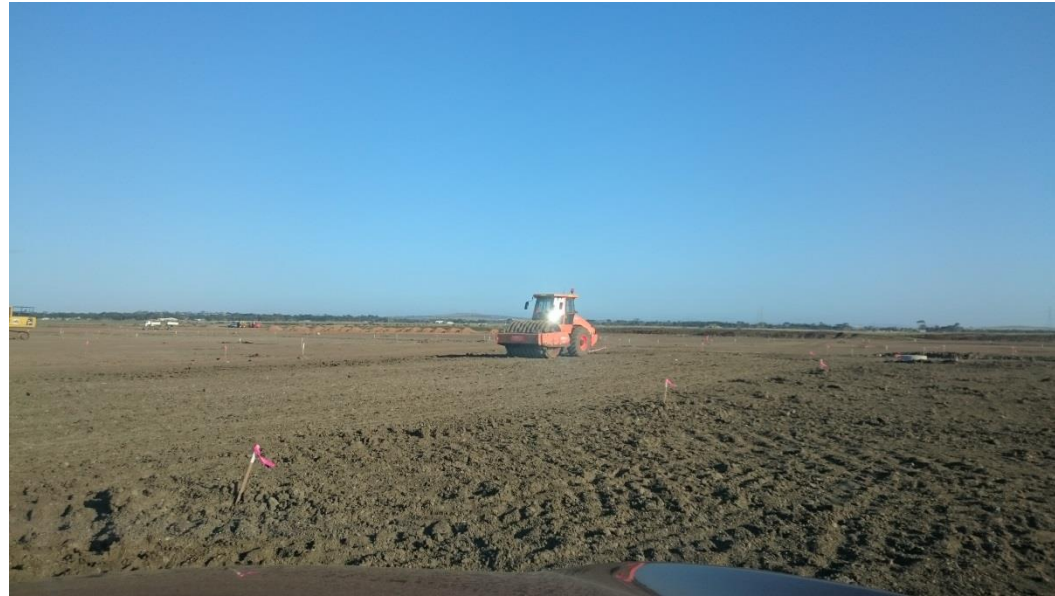
Stage 1: pad foot roller on layer 4 in grid I1 and I2
