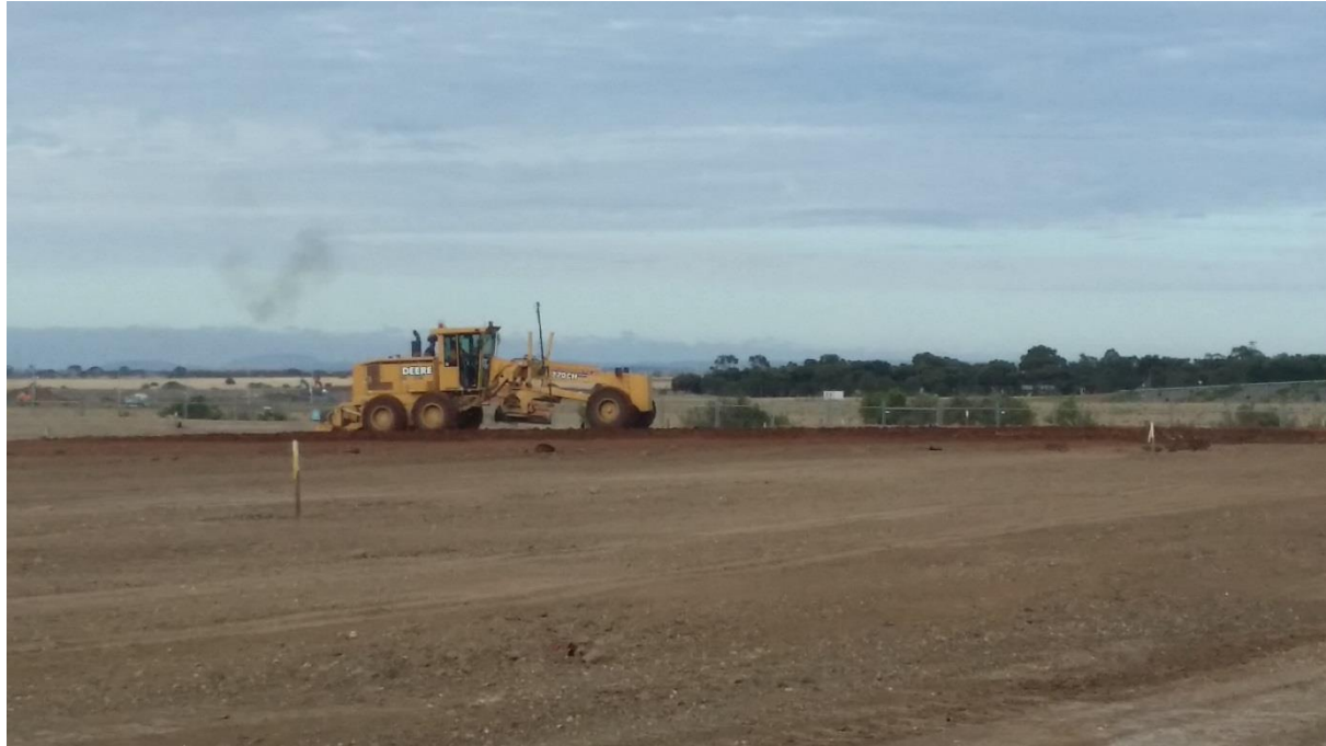
Stage 3: Scarifying of material in grid B5, B6, C5 (W) and C6 (W).
