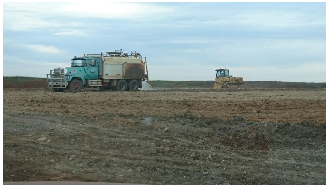
Stage 3: pad foot roller on layer 3 after being re-worked in grid E5, E6, F5, F6, G5 (W) and G6 (W)
