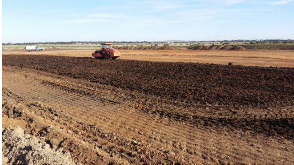
Padfoot Roller compacting layer 1 – E5 (east)/E6 (south-south-east)/F5 (west-north-west)/F6(west-south-west).
