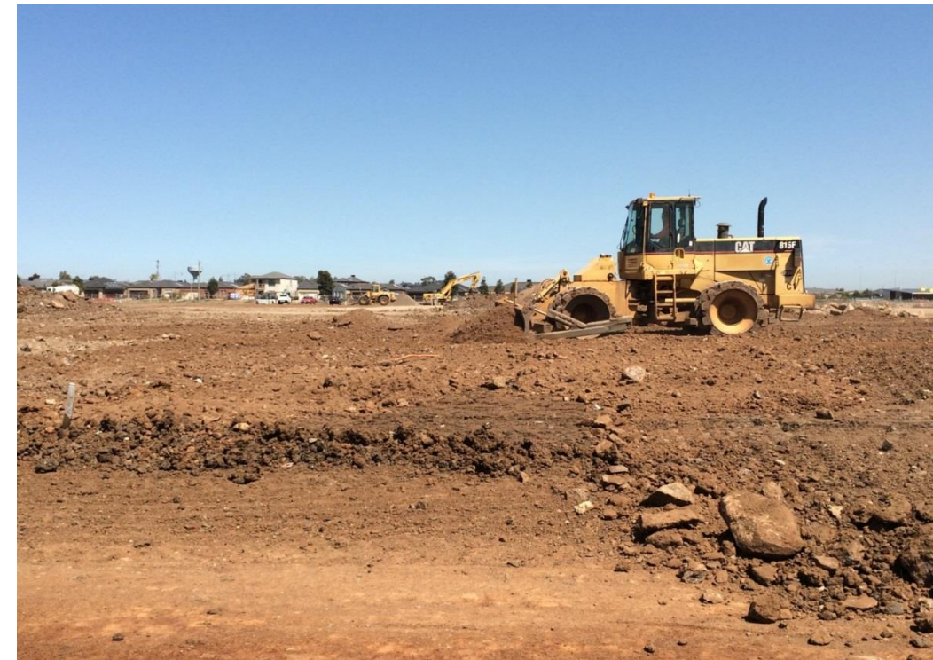
Compactor levelling the fill on grid layer D4-G4
