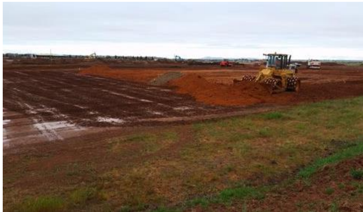
Compactor placing layer 1 – F6 (south)
