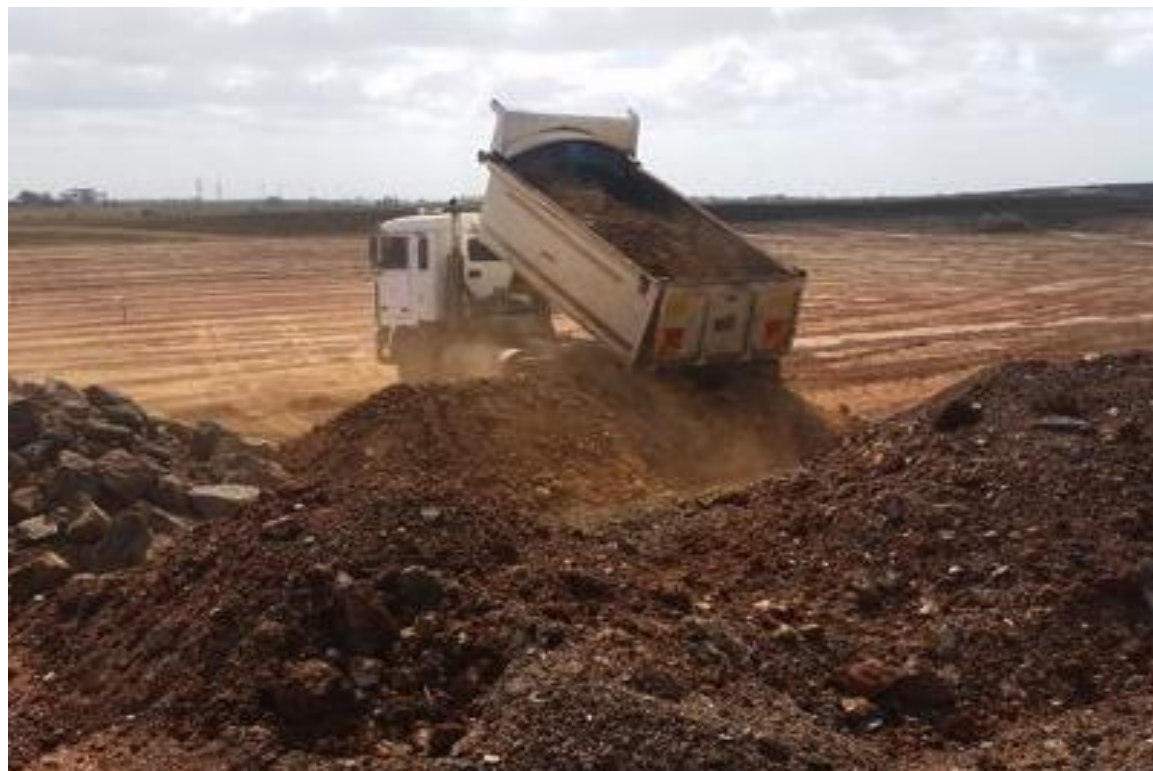
Dump truck unloading/stockpiling fill – E4 (west-north-west)
