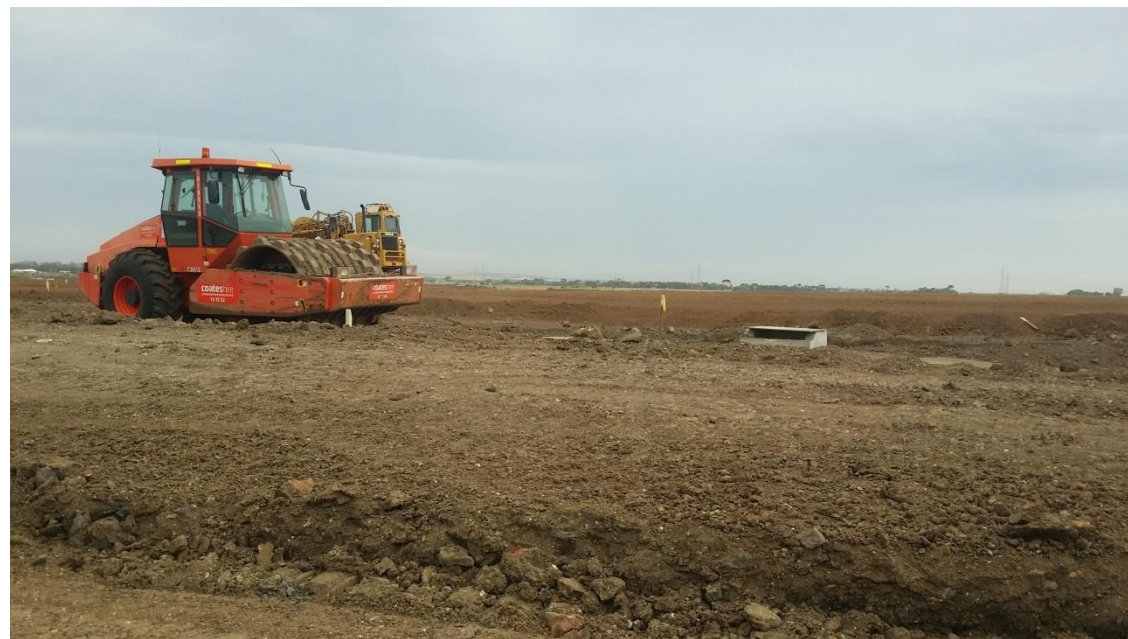
Stage 4: Placement and compaction of layer 1 material by CAT compactor in grid J5, J6 (S), K5 and K6 (S)
