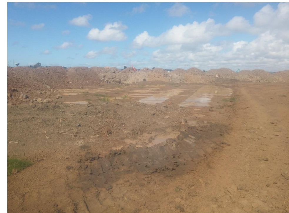
Image 3: Water pooling in grid H4
