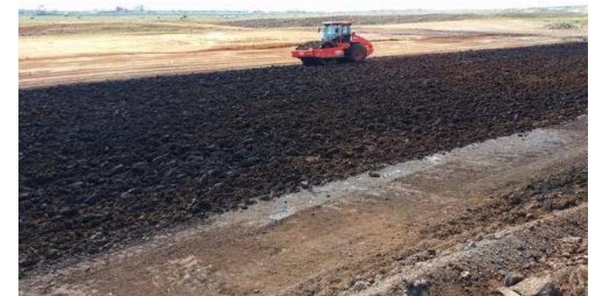
Padfoot Roller compacting layer 1 – E4 (north-north-east), F4 (north-north-east), and G4 (west-north-west).
