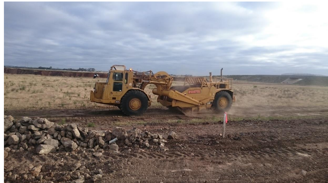
Stage 4: scraper removing topsoil layer as shown in Stage 4 site plan above
