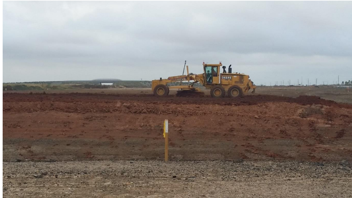
Stage 3: Scarifying of material in grid B5, B6, C5 (W) and C6 (W).
