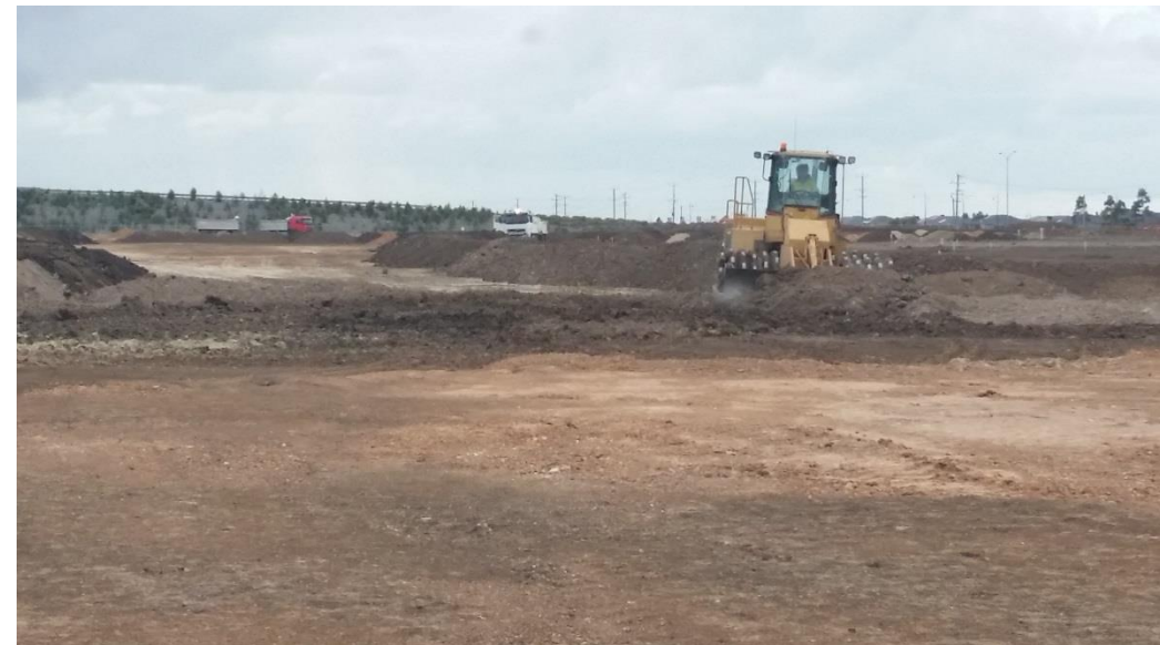
Stage 4: Placing of layer 2 in grid H5 (NE), H6 (SE), I5 (N) and I6 (S)
