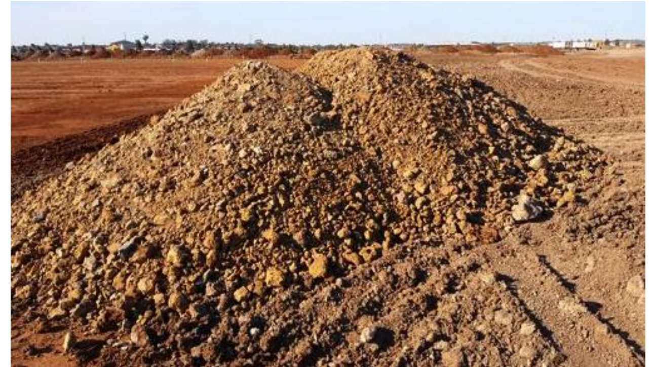
Stockpiled fill - column D
