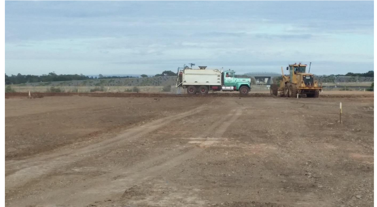
Stage 3: Moisture conditioning of scarified material in grid B5, B6, C5 (W) and C6 (W).
