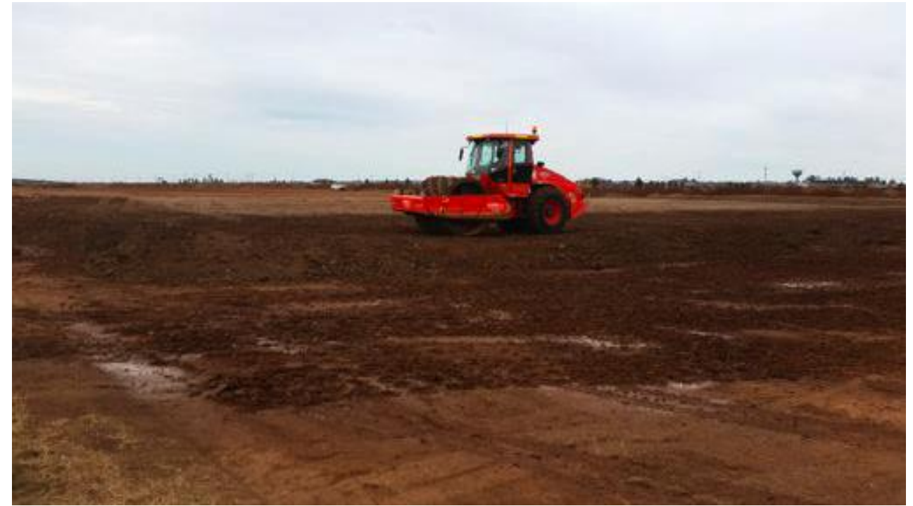
Pad-foot roller compacting layer 1 - grid column B
