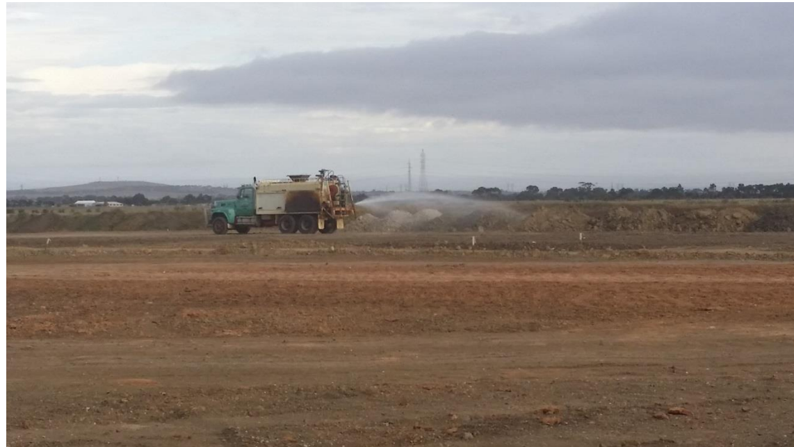
Stage 3: Moisture conditioning of stockpiled material in grid F5 and G5
