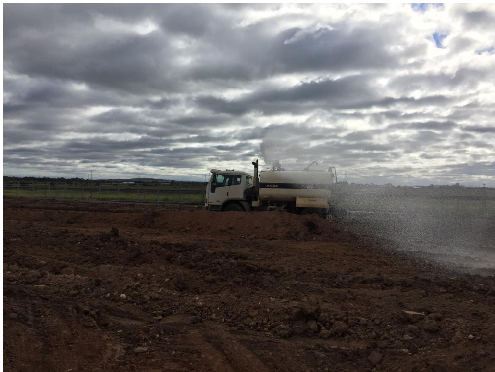
Stage 3: Moisture conditioning fill material prior to fill placement
