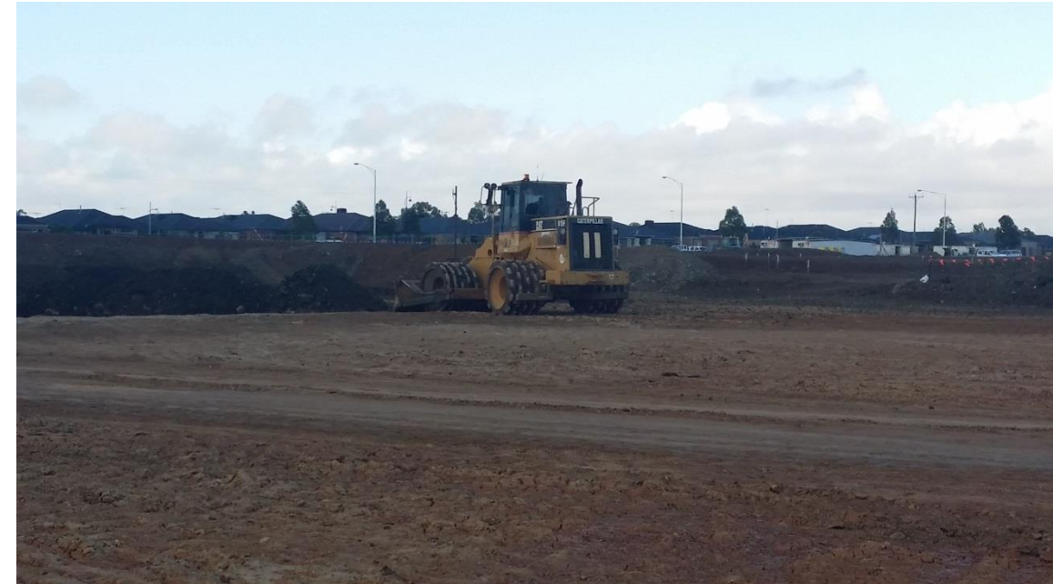
Stage 4: Placement of layer 1 in grid N2 (E) and O2.
