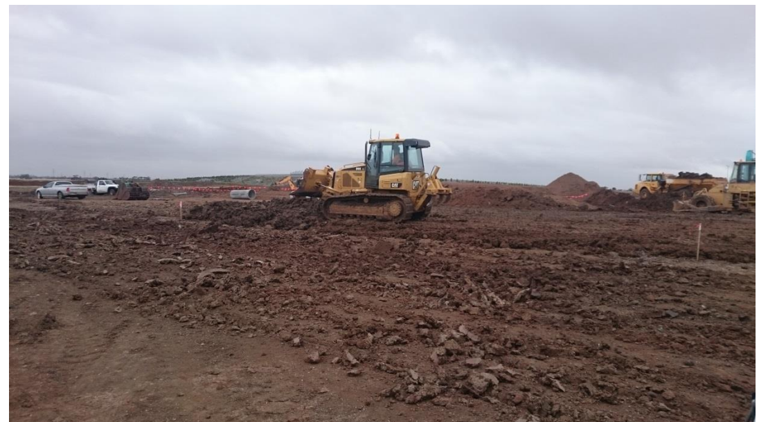
Stage 1: dozer placing material as part of layer 6 in grid K1 and K2
