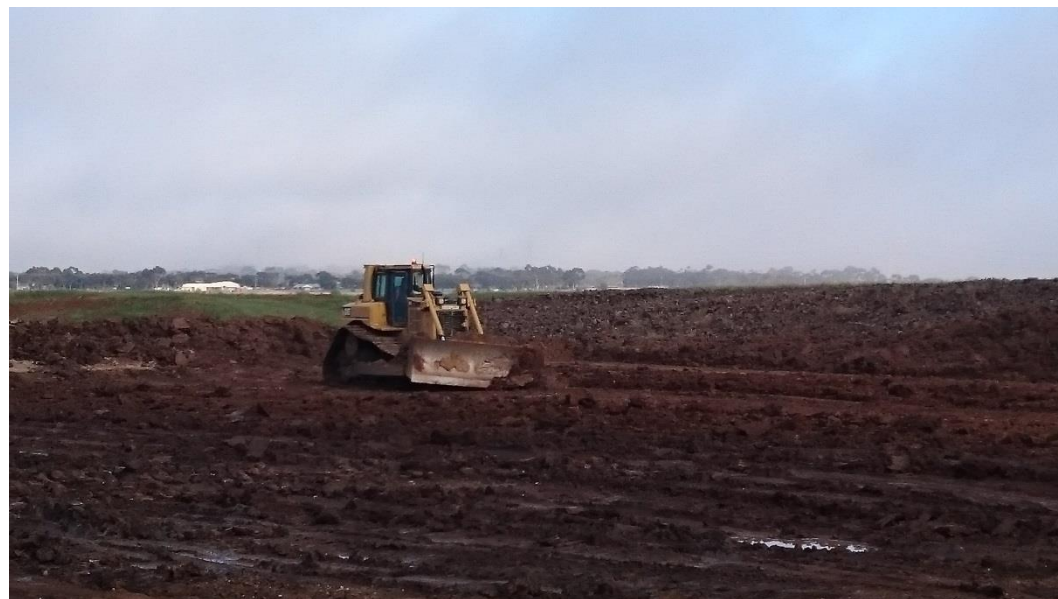
Stage 1: ripped layer 5 being moisture conditioned prior to placement of layer 6 in grid K2
