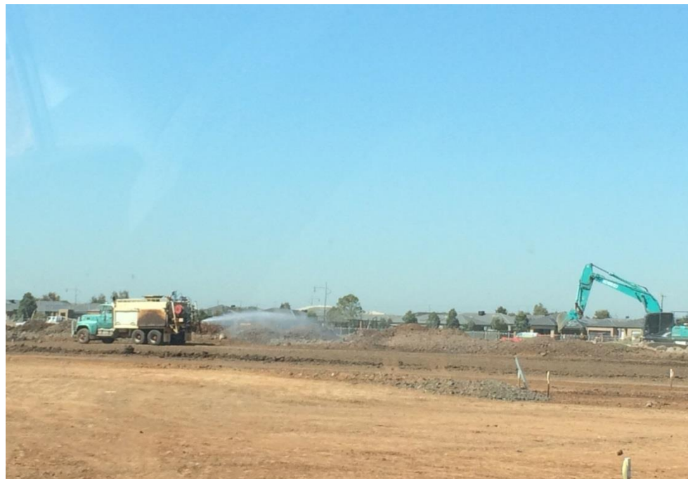
Water cart moisture conditioning grid layer D4-G4
