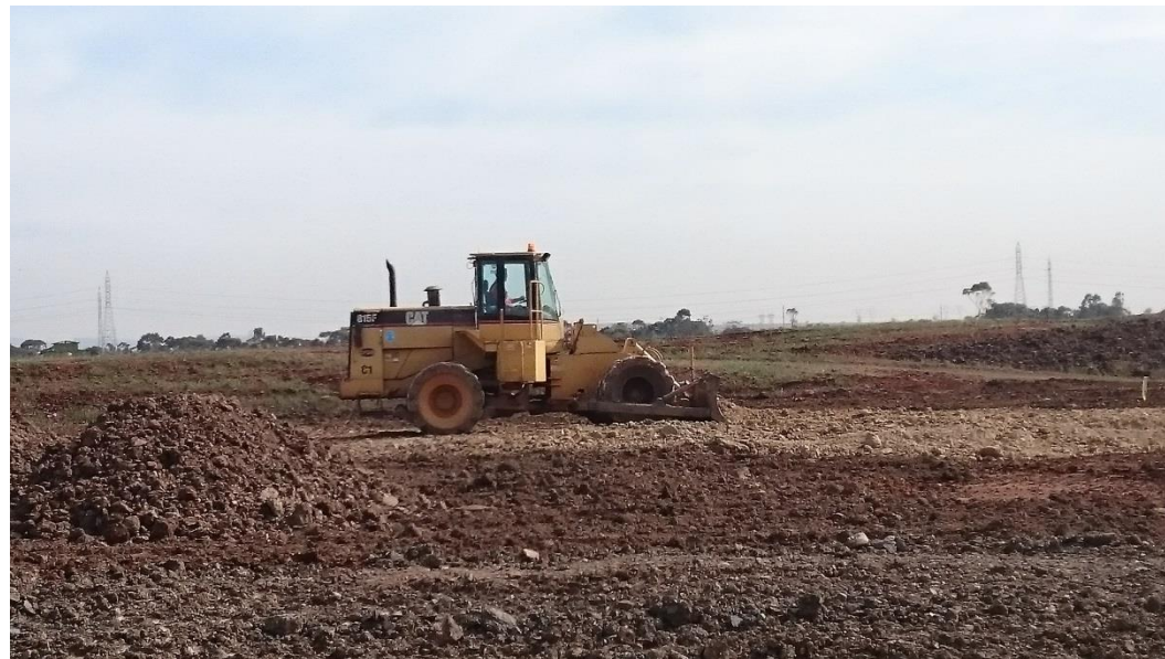
Compactor on layer 2 in grid F5, F6, G5 and G6
