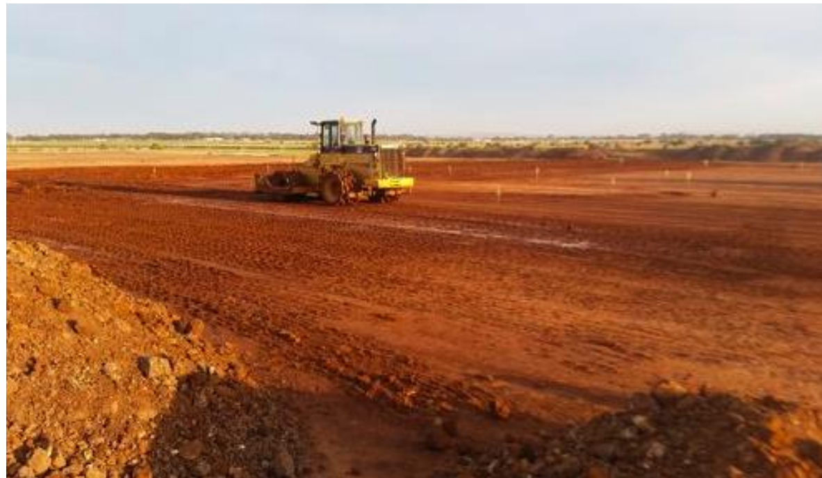
Compactor roughing-up/compacting subgrade – E4 (west-north-west)
