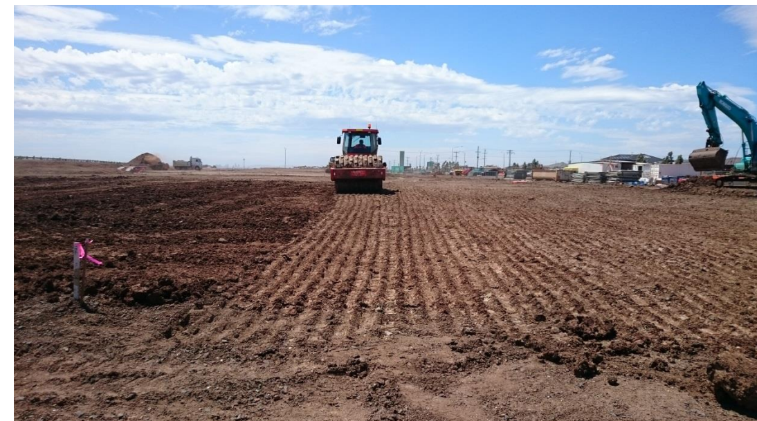
Stage 1: pad foot roller being used on layer 6 in grid K1
