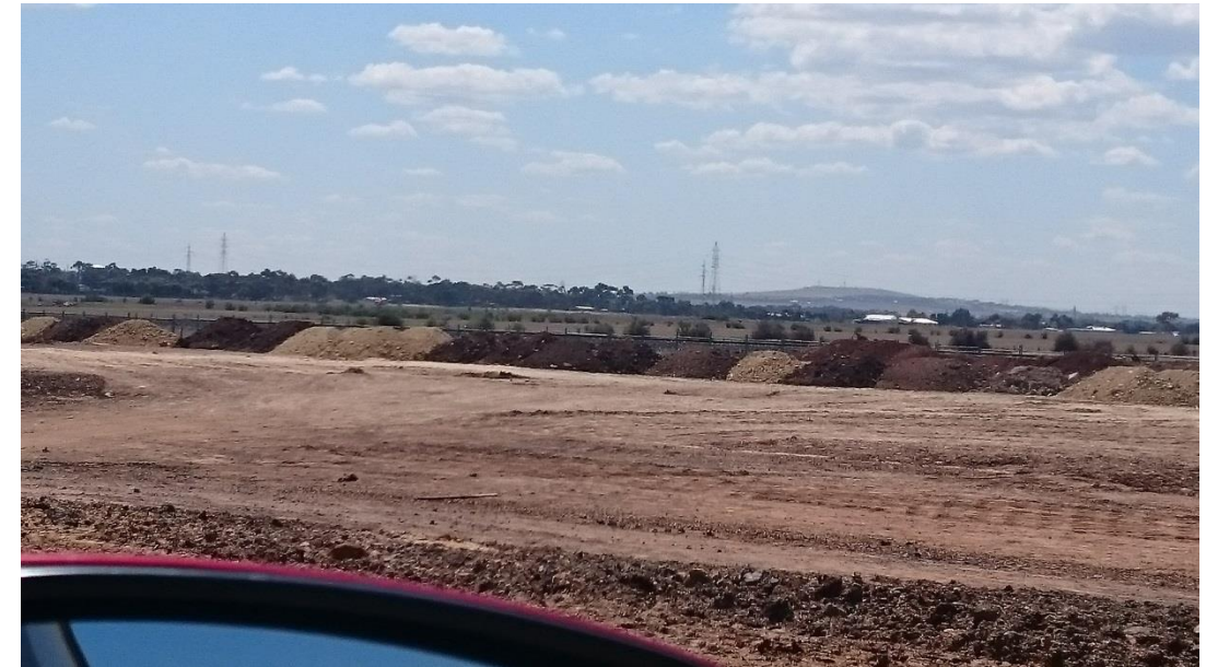
Stage 3: today's imported fill which has been stockpiled
