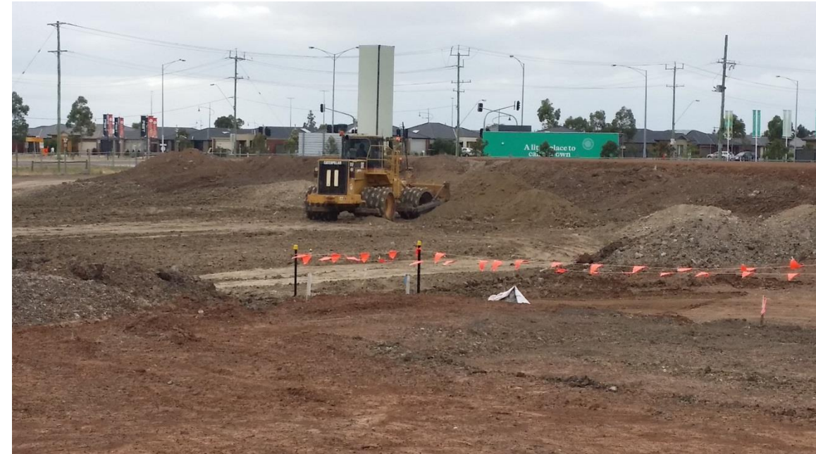
Stage 4: Further placement of layer 1 in grid N2 (E) and O2.
