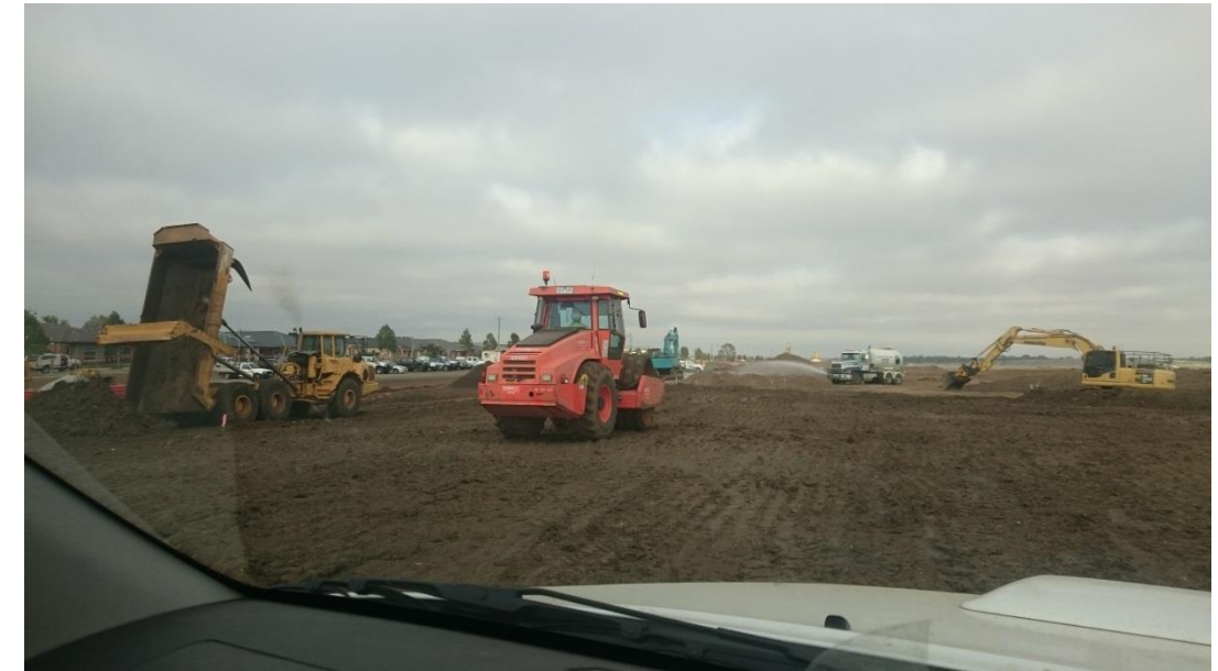
Stage 1: pad foot roller used on layer 7 in grid N1
