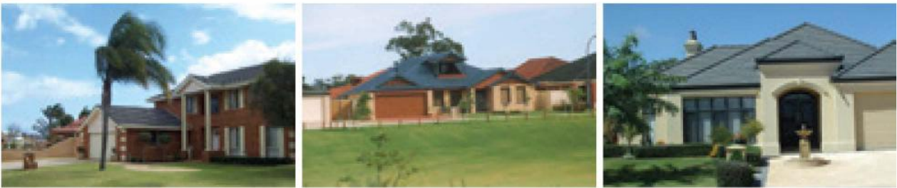
Dark roofs are exhibited. Colours are incompatible with 'Touch of White' colour palette.
