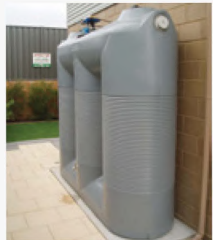
Example of the rainwater tank.
