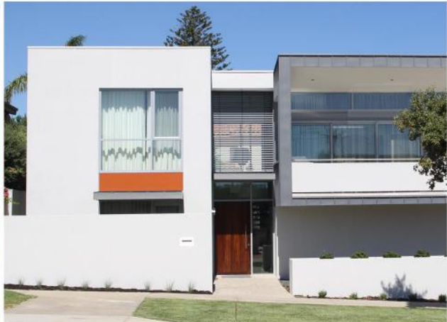
White walls offset by feature colour, natural timber door and zinc cladding.
