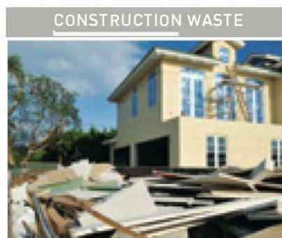
Onsite separation of wastes for recycling or reuse. (Source: Zero Waste WA)
