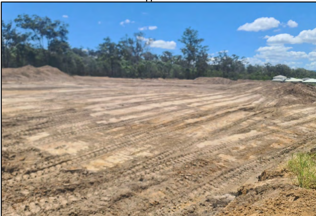
Picture 1: Stripped Natural Surface
