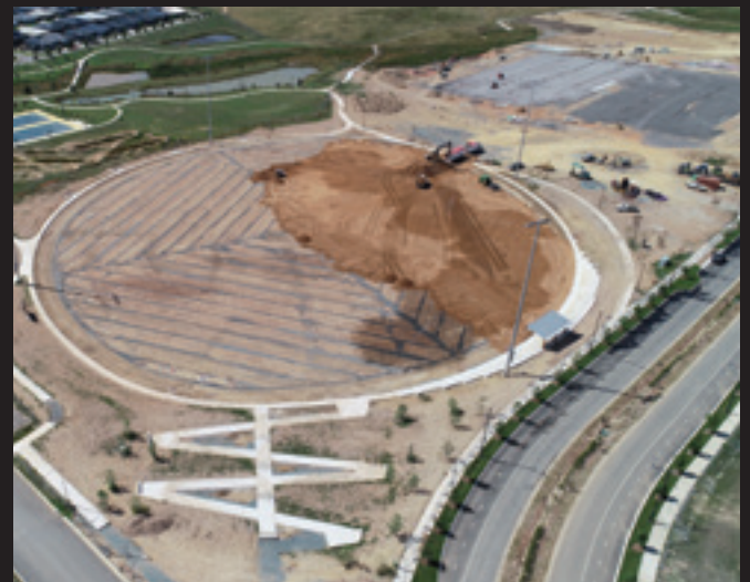
↑ Image: Sports Field 3 and 4 construction.
