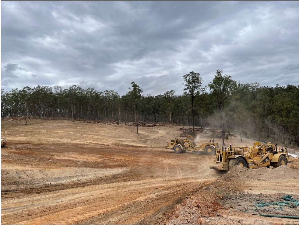
Figure 1 – Scrapers running circuits placing and spreading fill material. (Taken 25.11.2020)
