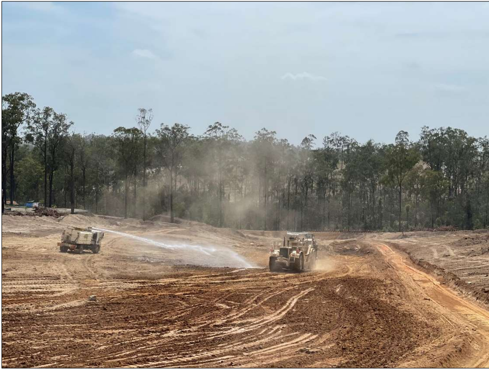
Figure 3 – Scrapers running circuits with a water truck adding moisture. (Taken 30.11.2020)
