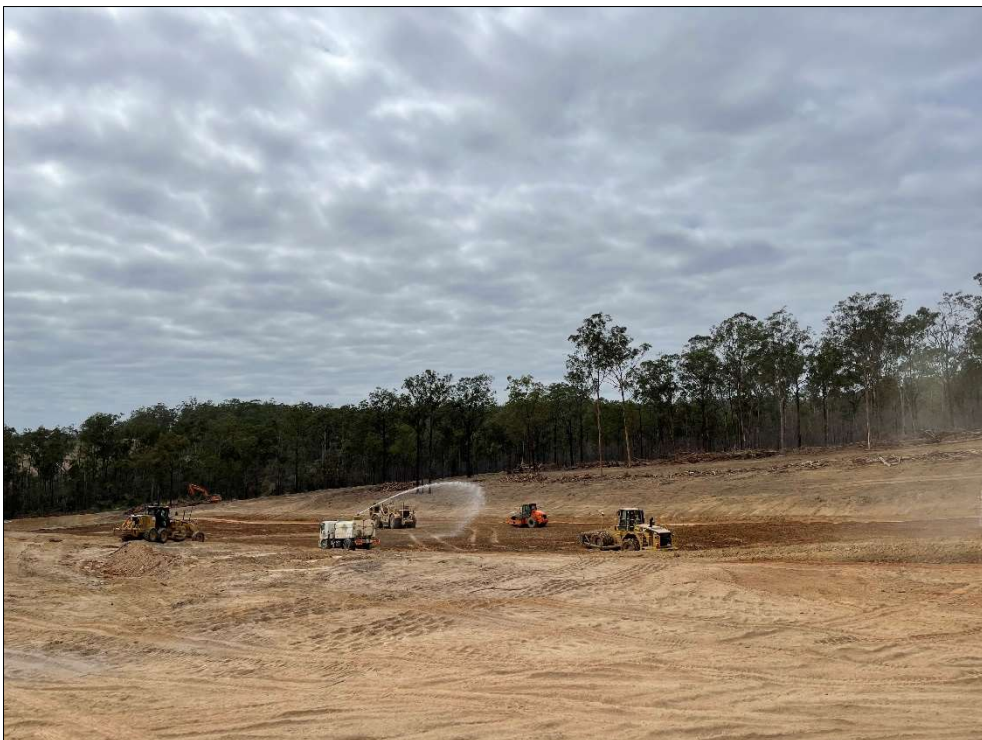
Figure 4 Heavy machinery used throughout bulk earthwork activities. (Taken 1.12.2020)
