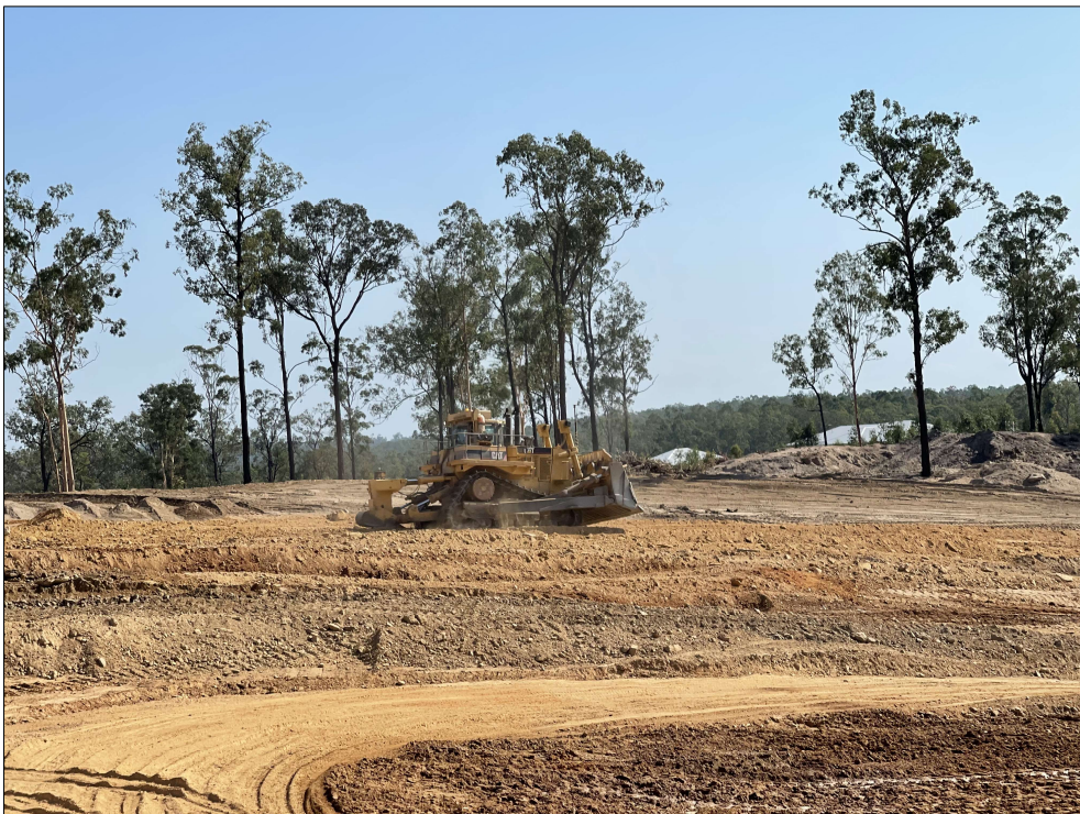
Figure 6. Dozer spreading and placing fill materials on house lots. (Taken 02.12.2020)
