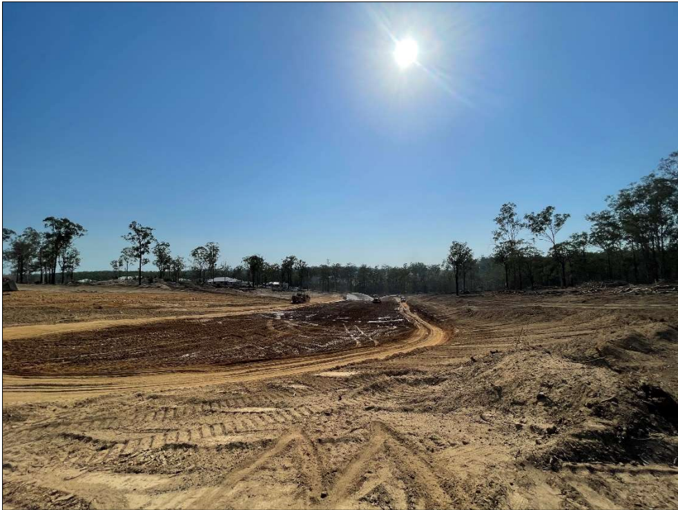
Figure 5 – Water cart used to moisture condition the fill material placed. (Taken 2.12.2020)
