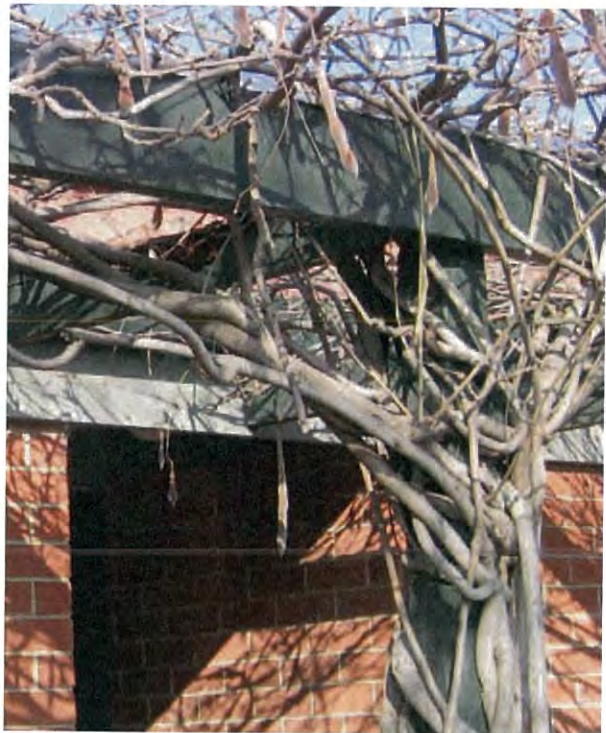
Vines and creepers act as ladder fuels.
