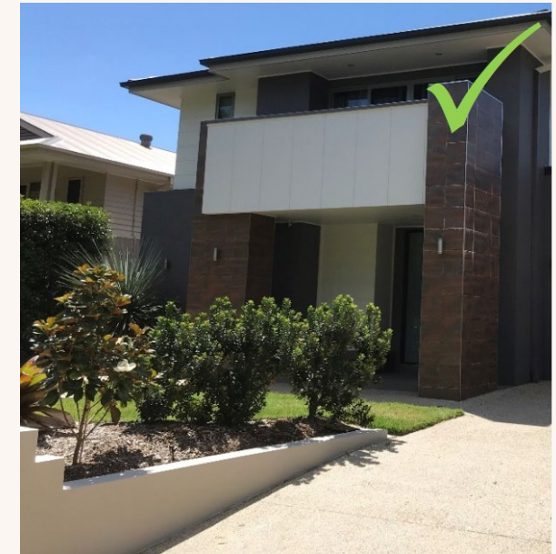
White rendered masonry retaining walls are acceptable.
