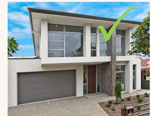
An example of a low profile roof with wide eaves and a modern architectural gutter.
