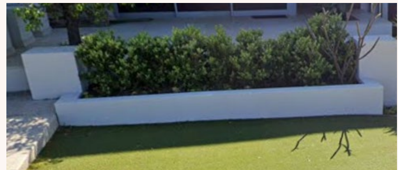
An example of a white rendered masonry wall.
